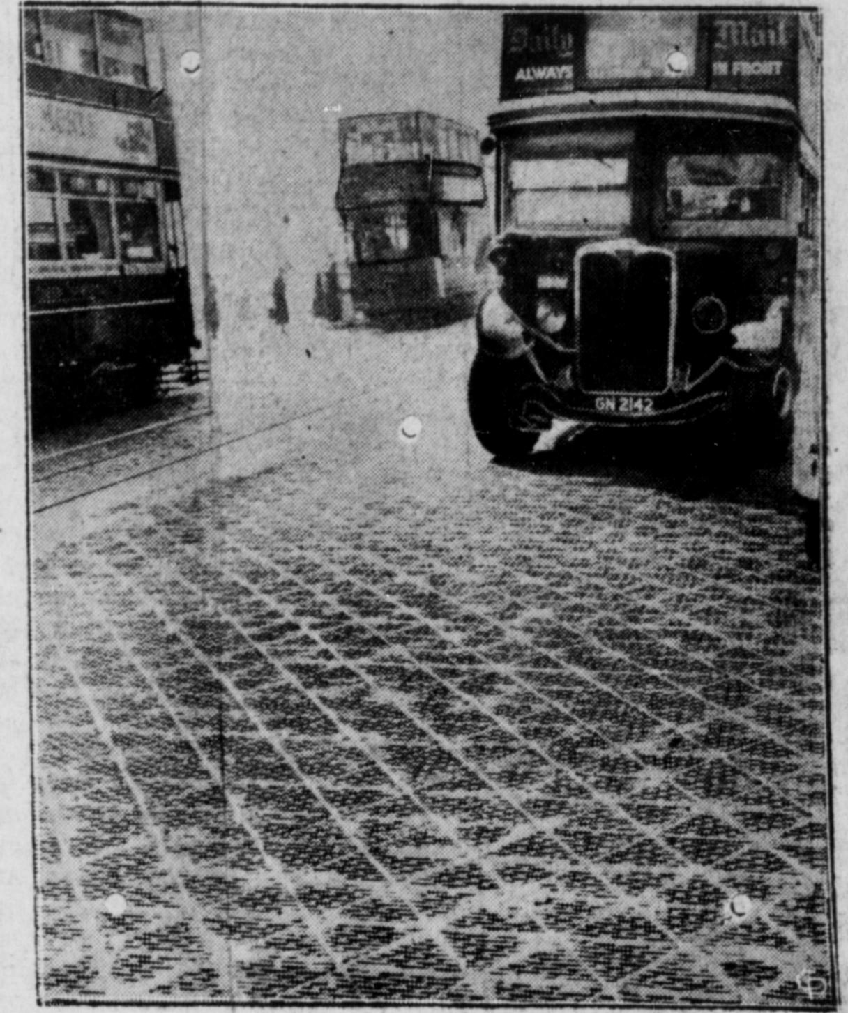
That section of Upper Street in Islington Borough, London, whereon corrugated iron street paving is being tested, is pictured. The corrugations, designed much after the style of the familiar auto tire treads, are expected to reduce skidding to the ultimate minimum, and London traffic authorities are expectant in the matter of the wearing quality of the road. They believe that in this case, surely, the familiar guarantee to "wear like iron" will
