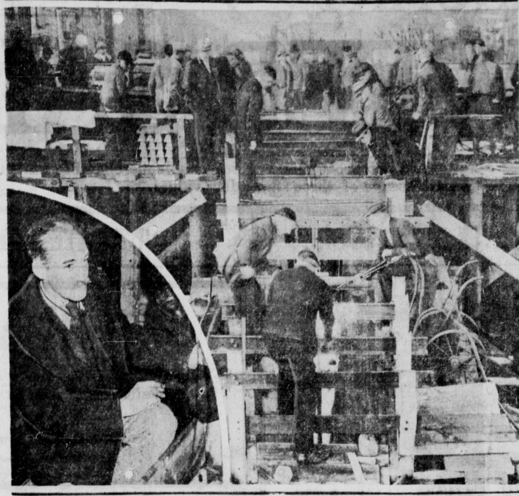
The first step in construction of the new sloop that Harold S. Vanderbilt will offer as defender of America's Cup next summer against the British "Endeavor II" is shown as the keel was poured at Bath, Maine. The \$300,000 craft will have a "fin" of lead weighing between eighty and ninety tons. In the lower left is W. Starling Burgess, designer, watching start of construction.
