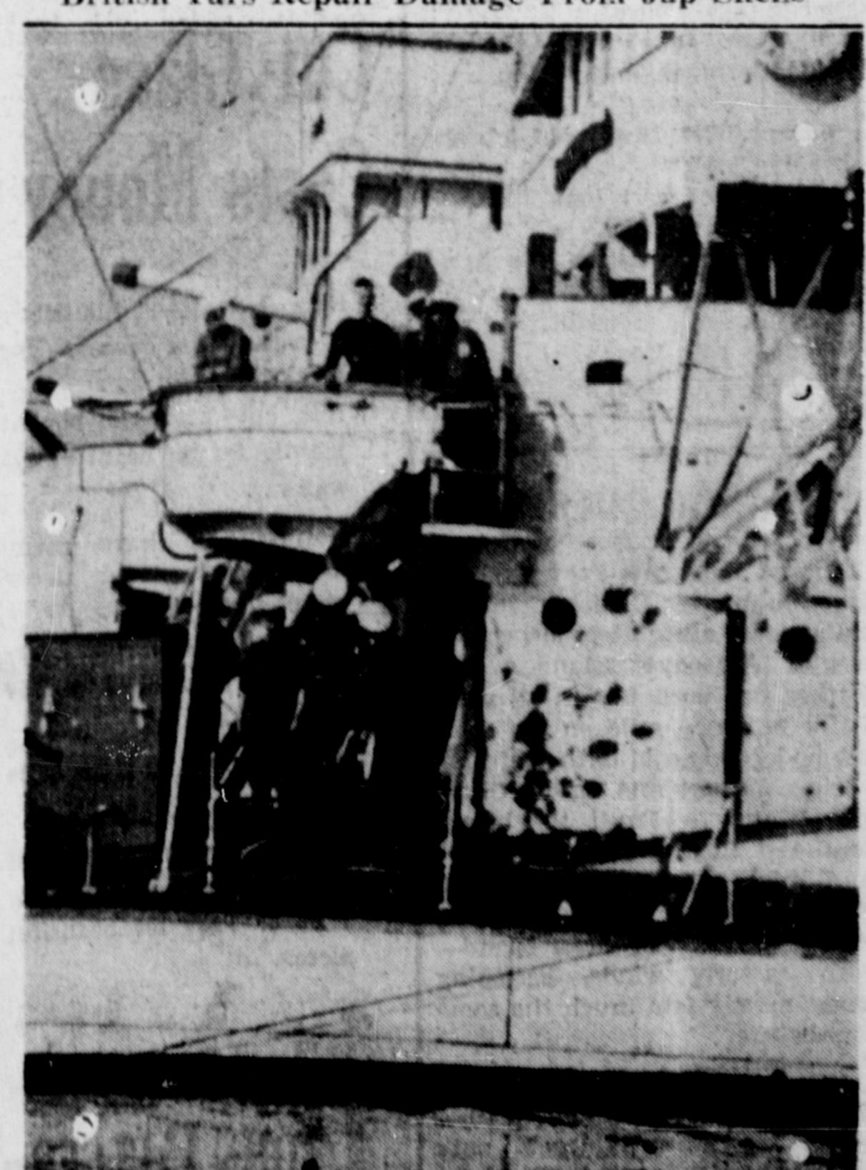
Seamen of the British gunboat Ladybird upon arrival at Shanghai are pictured repairing damage done to the vessel when it was attacked by Japanese bombing aeroplanes on the Yangtse some time ago. The tars found it necessary to plug a hole in the boat's hull down near the waterline. In this picture they are removing traces of shelling from the upper structure.
