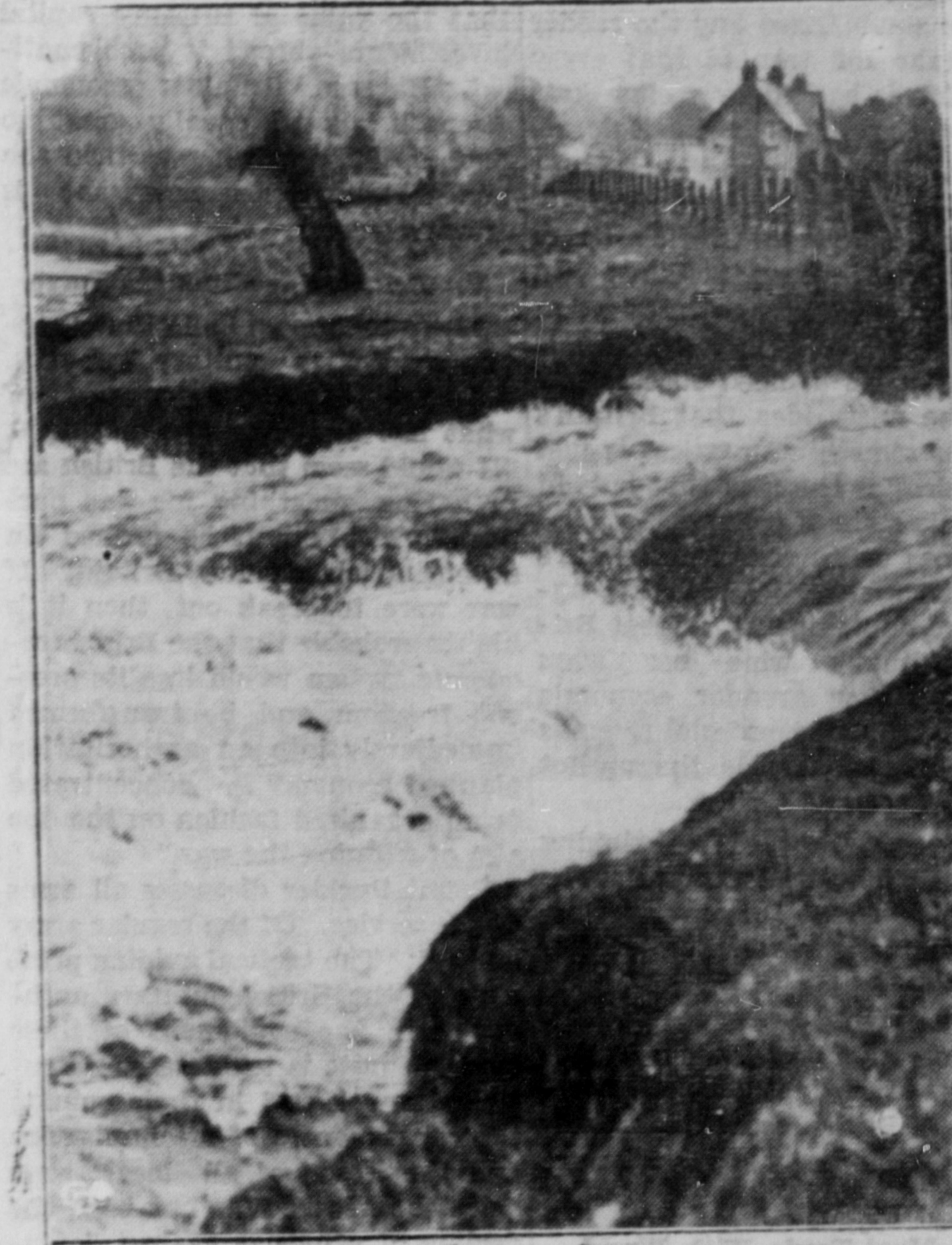
The Lagan River in the Belfast district of Ireland, pictured as it broke through the embankment at the Stranmillis Lock. As a result of torrential rains the river rose to a height unprecedented for the last 50 years and despite the fact that all sluices had been lifted to give the water speedy clearance this gap approximating 15 yards was made in the embankment.
