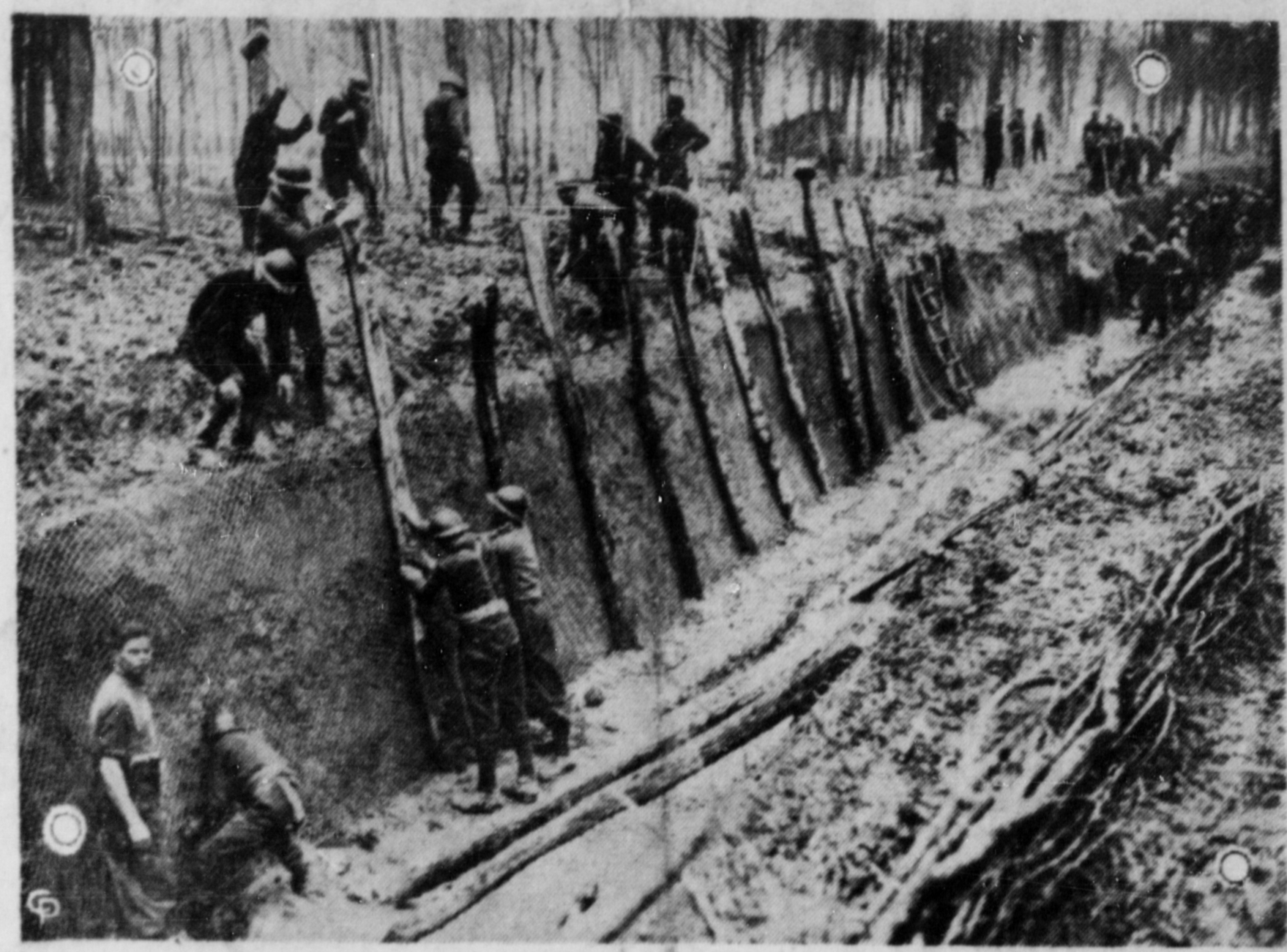
French engineers are shown at work on one of the gigantic ditches they have constructed along the Western Front as a barricade against German tanks. The ditches are dug with steep walls that give a tank a drop of about 15 feet and make them easy prey for the anti-tank guns.
