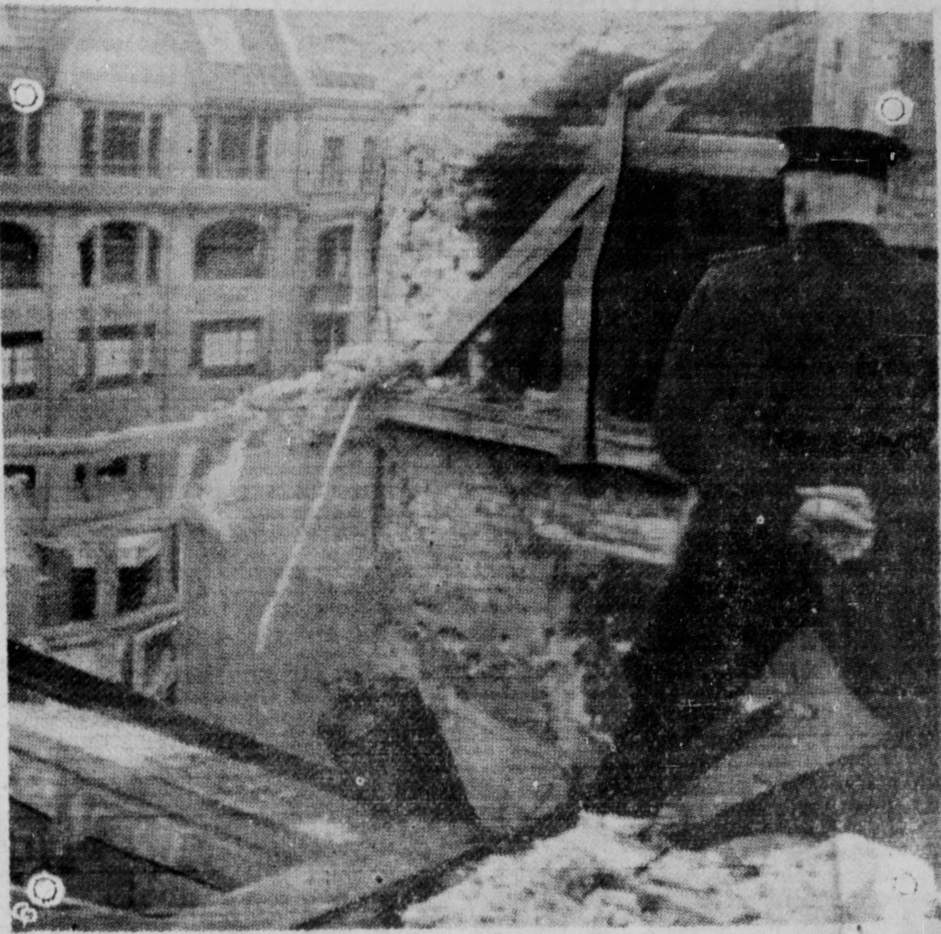
A German fireman looks into the wreckage of a building on Kottbuser Strasse, Berlin, less than two miles from Wilhelmstrasse, where German government buildings are located. This building and others in the vicinity were bombed by British airmen retaliating for German bombings of London.
