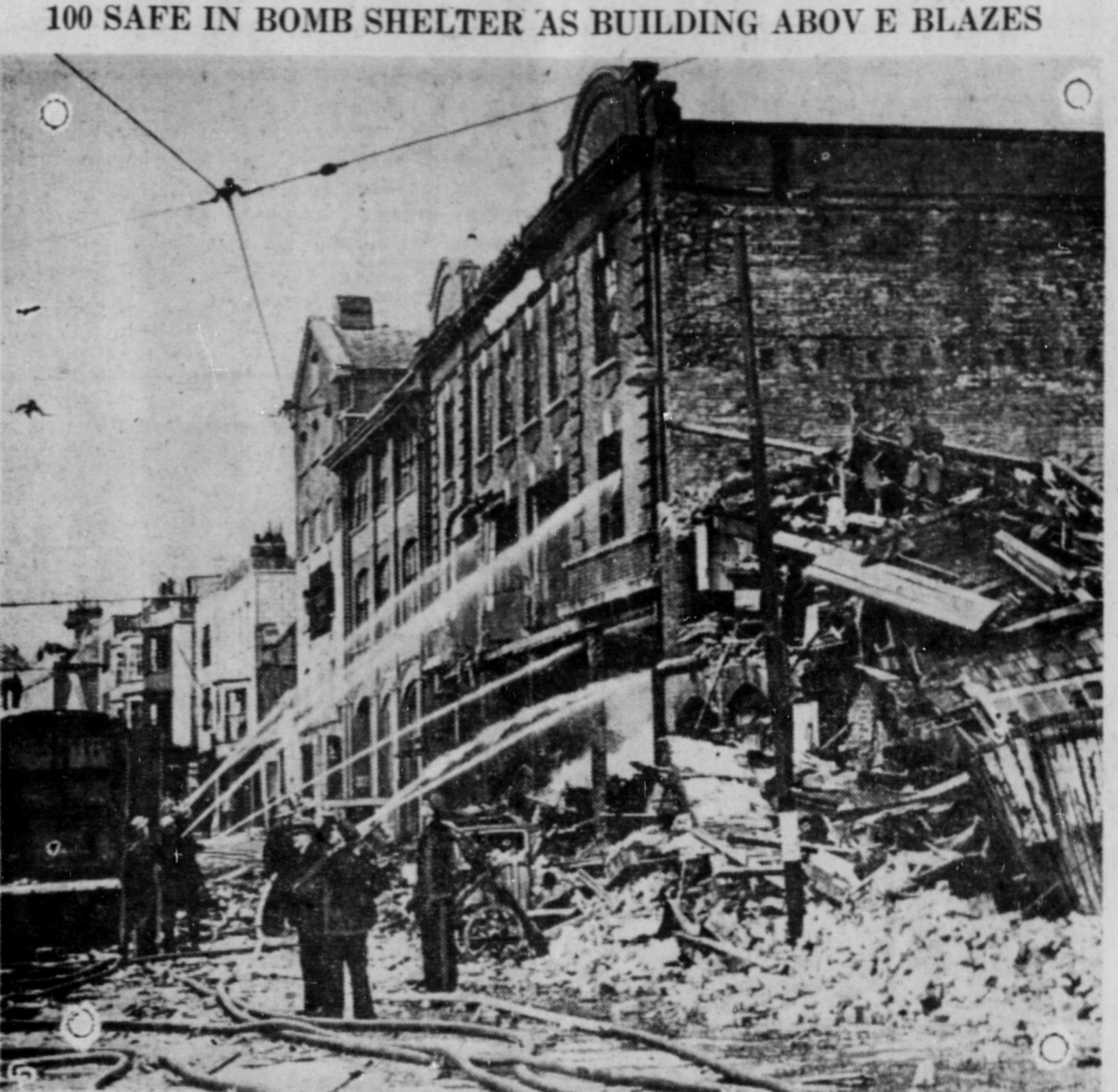
100 SAFE IN BOMB SHELTER AS BUILDING ABOVE BLAZES The earth rumbled and some of the 100 refugees in the bomb shelter moved uneasily, but the rumbling stopped and no one was hurt in the shelter itself at Southampton, England. Immediately above the shelter, however, this furniture depository caught fire from Nazi-dropped incendiary bombs and the local firemen are shown quelling the flames.
