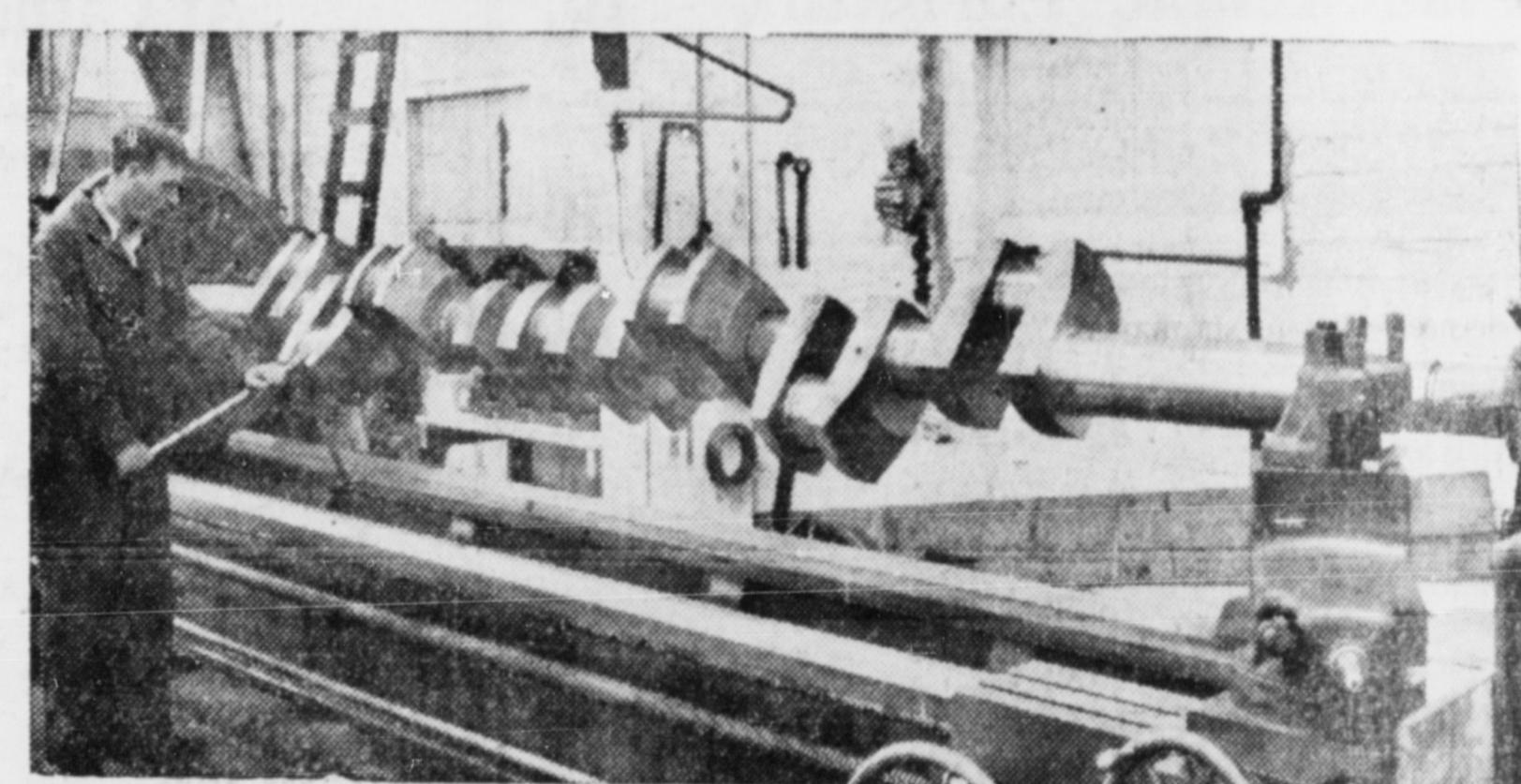
The huge shaft of a marine engine gets final adjustments on a giant lathe in a C plant. Enormous in size, the shaft is as crooked as a cork-screw, yet crooked with complet symmetry. It must be milled and polished until the slightest pressure from one of the cylinder heads will start it revolving when the motor is started up.
