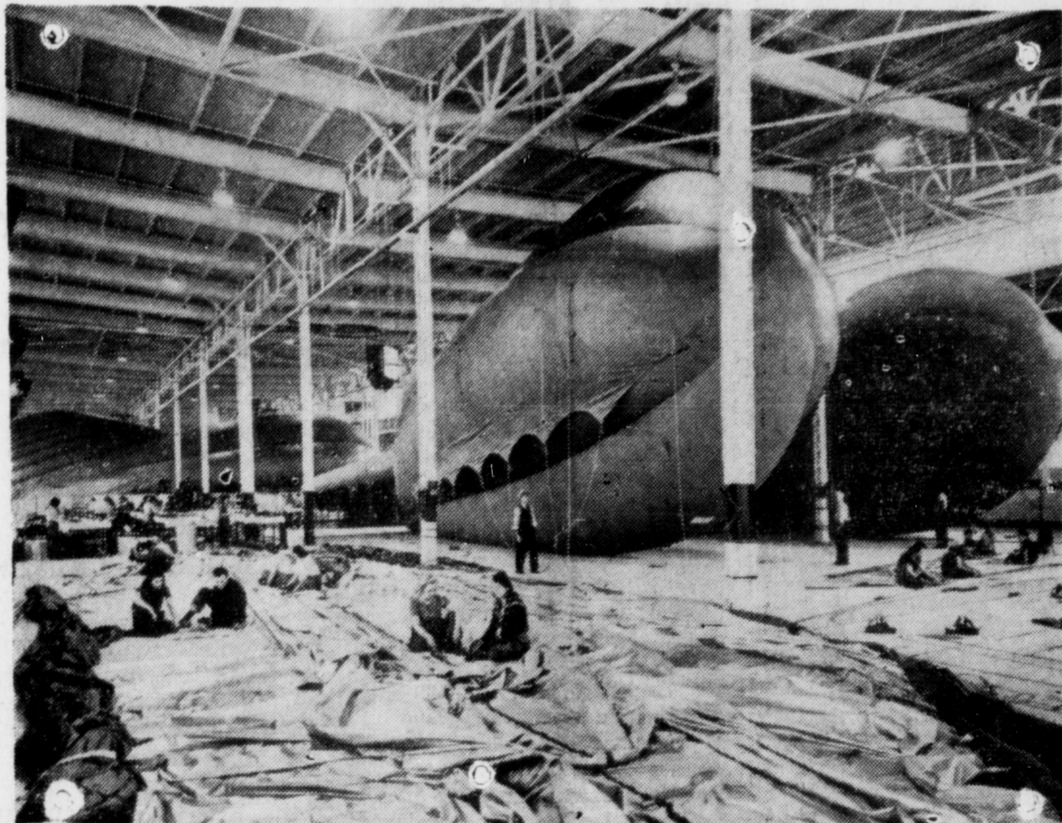
A view of the new huge balloon room at the plant of the Firestone Tire and Rubber Co. in Akron, O., where as many as 12 great barrage balloons may be inflated at one time. The company is going into mass production of these gas bags that proved their worth in defending vital points against marauding aircraft in Britain. Workers in foreground are assembling big bag. The inflated balloons in rear have passed inspection.
