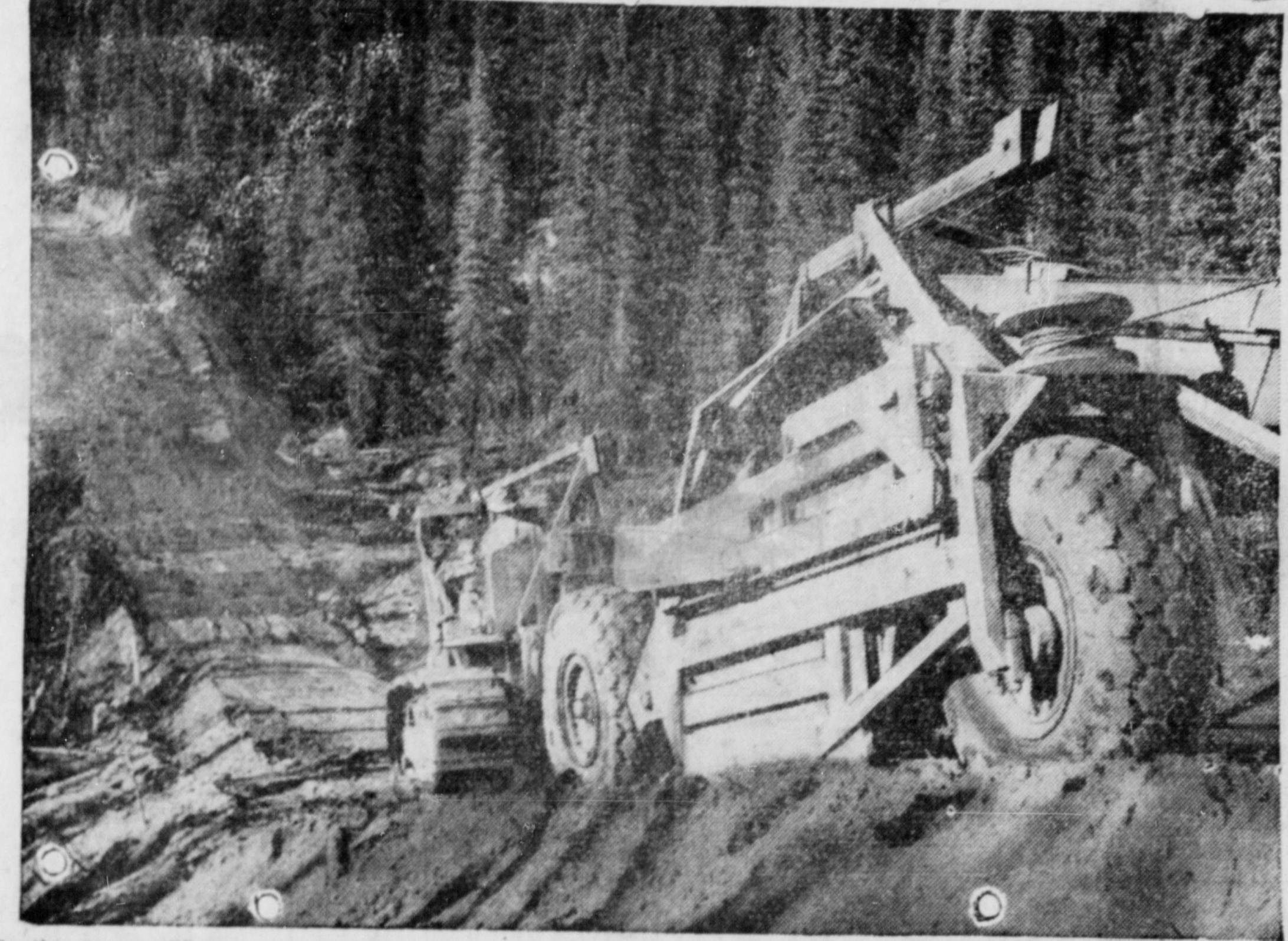
On this "carry-all" tons of earth are moved from one section of years old. When muskeg is removed the ice melts, creating heavy of the road to a fill. Hidden two or three feet under the muskeg morass. U.S. Army engineers have solved the problem. Bishop G. in some sections along the road are glacial ice formations thousands A. Rix tells of work on the Alaska in an interview published today.
