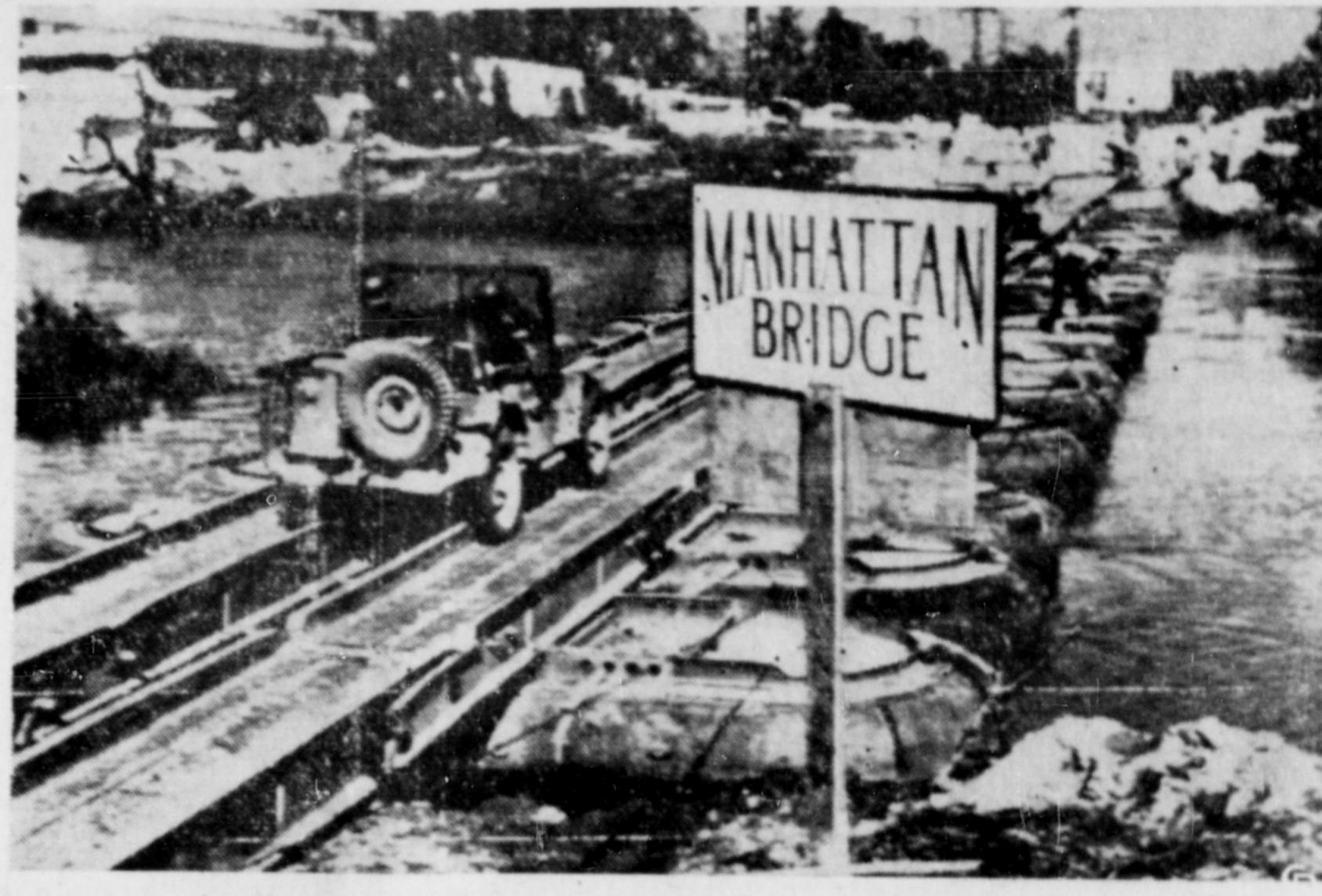
This pontoon bridge over the Volutrno river in Italy is named for the bridge over the East river in New York. The bridge is east of Dragoni and is replaces the stone bridge demollished by retreating Nazis, part of which may be seen at left.
