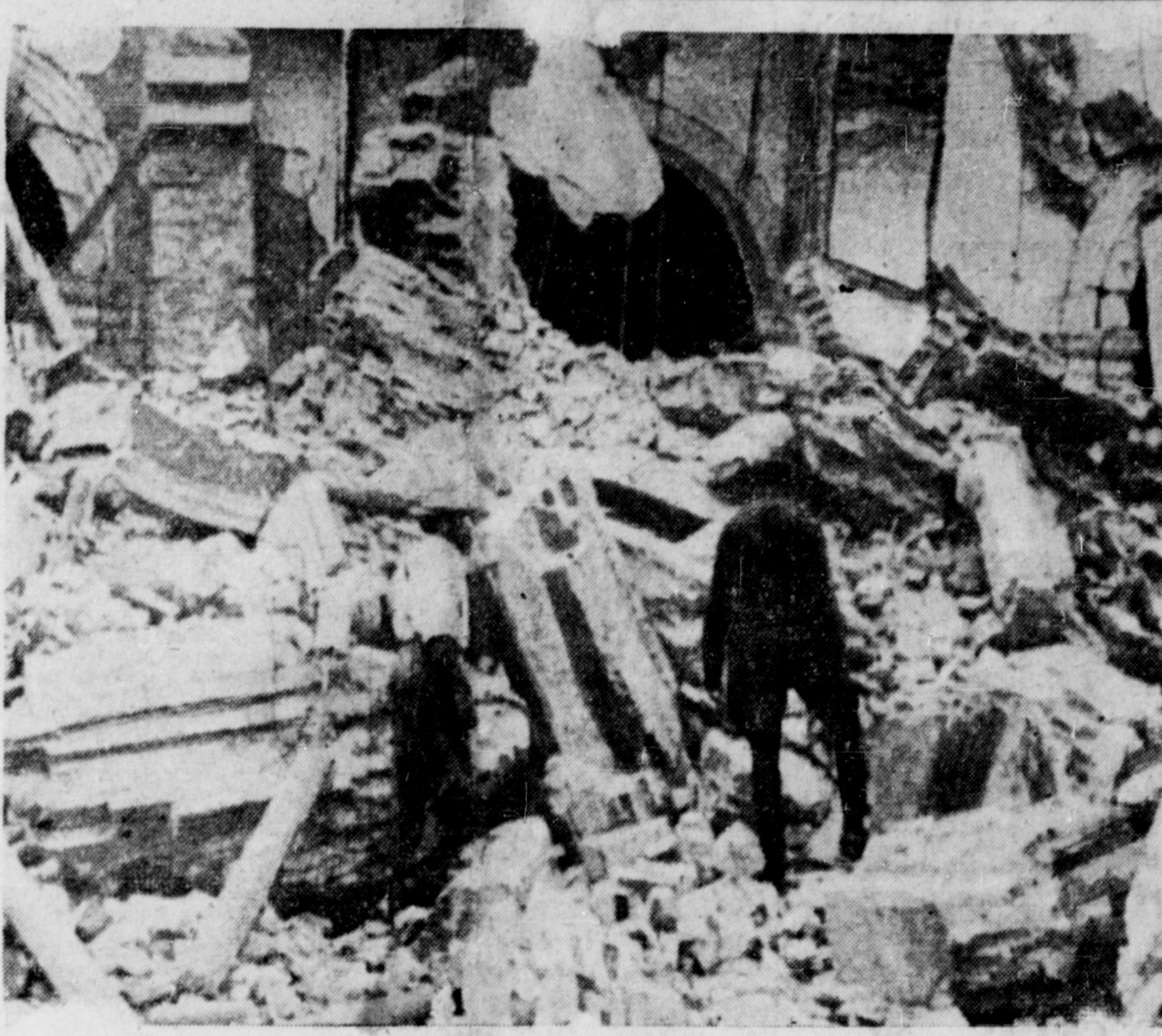
QUAKE VICTIMS SEARCH DEBRIS FOR BELONGINGS —The city of Matanzas, on the north-east coast of the Dominican republic, felt the full force of the devastating earthquake and tidal wave which hit the country. Residents are shown combing the ruins seeking their belongings after the first shock. Most of the inhabitants had fled to safer areas fearing a recurrence of the disaster. Many of the buildings which withstood the first shock, crumbled during the 40-second tremor which rocked the city.
