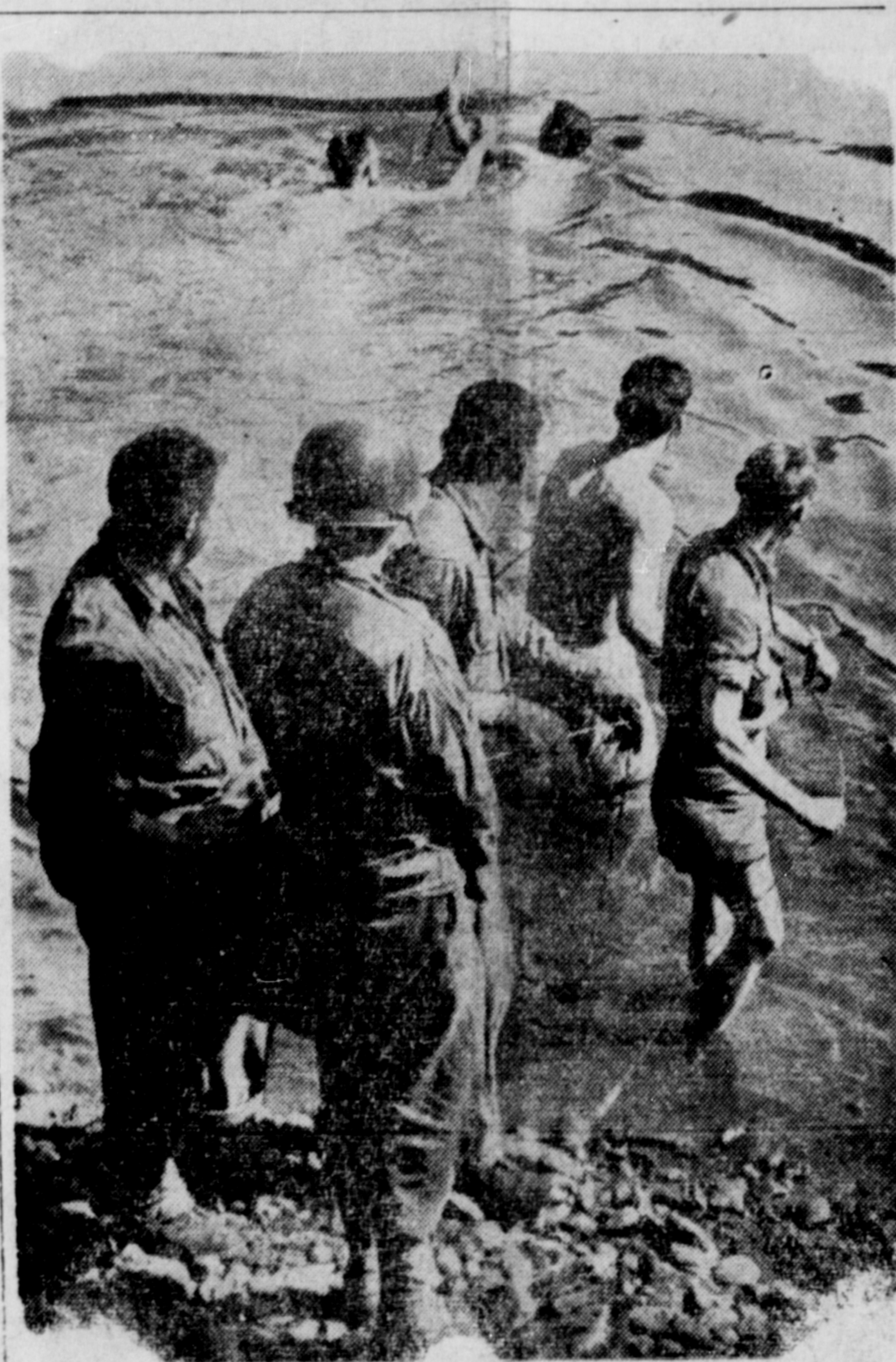
SWIM LINES ACROSS MOSELLE—Three times, the vital communication lines laid across the Moselle River in France by a signal battalion were broken. This time, the men, determined to get across, decided to swim the lines across farther down the river. Two of the men can be seen in the water holding the end of the cable as they swim across, while others of the unit stand on shore feeding the cable to them.
