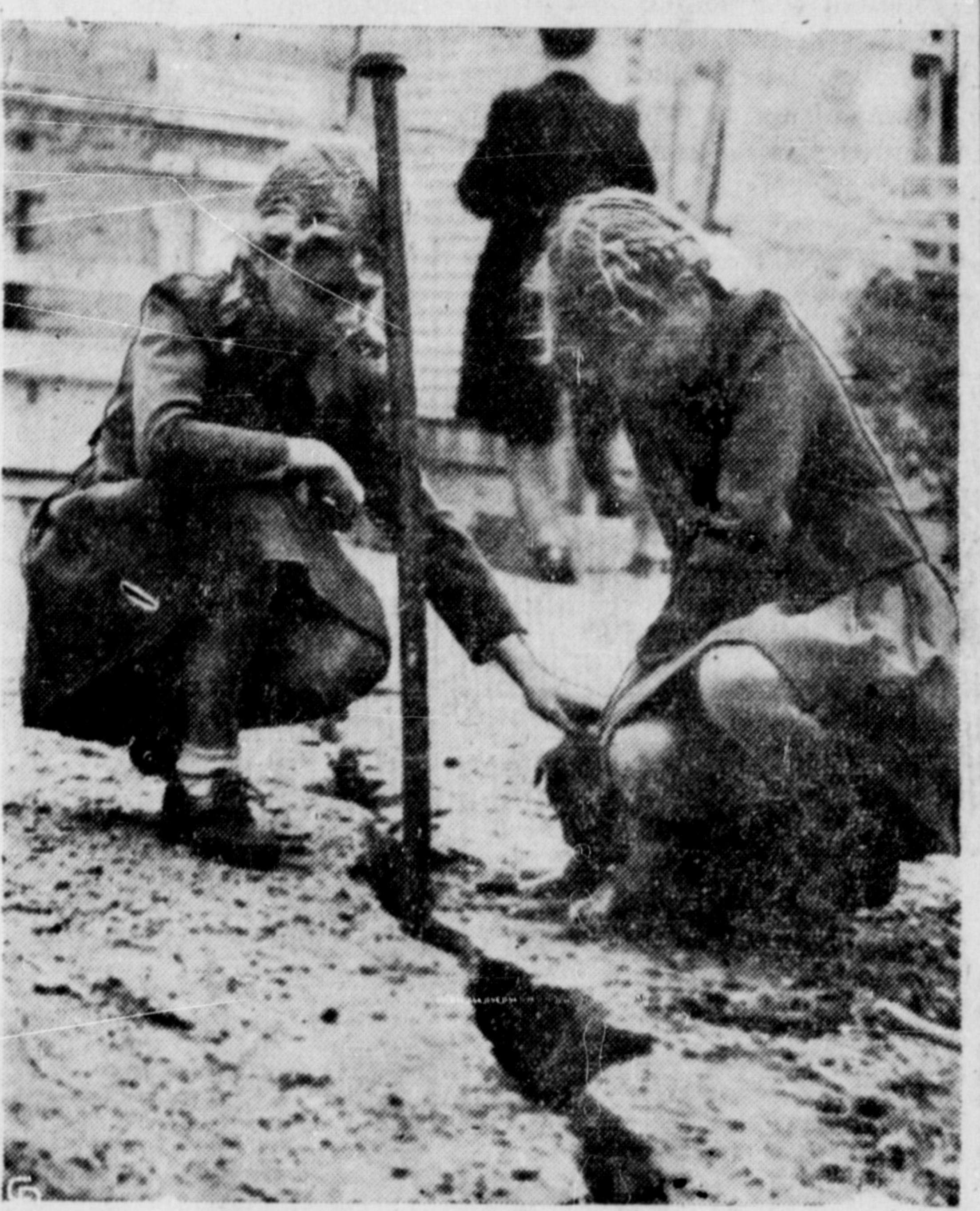
MINE CAVE-IN INDUCES EARTHQUAKE —When tunnels in a coal mine collapsed in East Lithgow, Australia, the town came close to panic as houses rocked and cracks appeared in the ground, giving all the evidence of a severe earthquake. Here, two young girls push a six-foot crowbar into a fissure that appeared in their backyard.
