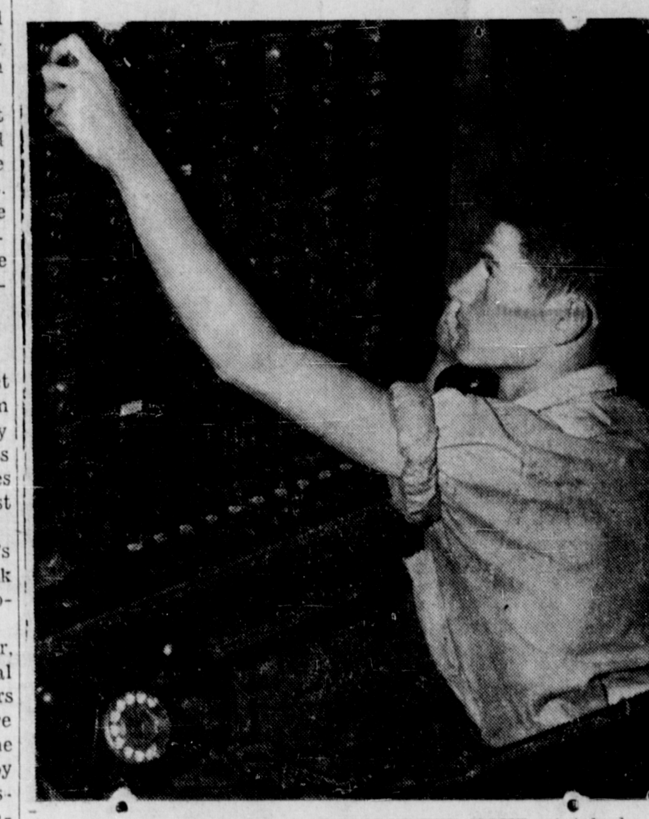
"WARRIOR" CAN HANDLE 250 CALLS PER HOUR—A telephone exchange which could adequately serve the needs of a fair-sized town is the nerve centre of the internal communications system on board the Canadian aircraft carrier "Warrior." The main telephone exchange has 138 lines and nine of those are party lines with one or more extensions. During daylight hours at sea, it usually handles about 250 calls an hour, while in port the number rises to around 400. In addition to phones on the exchange, there are 45 direct lines between operational centres and 108 lines leading to Damage Control headquarters. Also there is a public address system audible anywhere in the ship. At the switchboard of the main telephone exchange in this picture is Able Seaman Louis Vernerey of Saskatoon, Sask., one of the four seamen of the torpedo branch who operate the switchboard.
