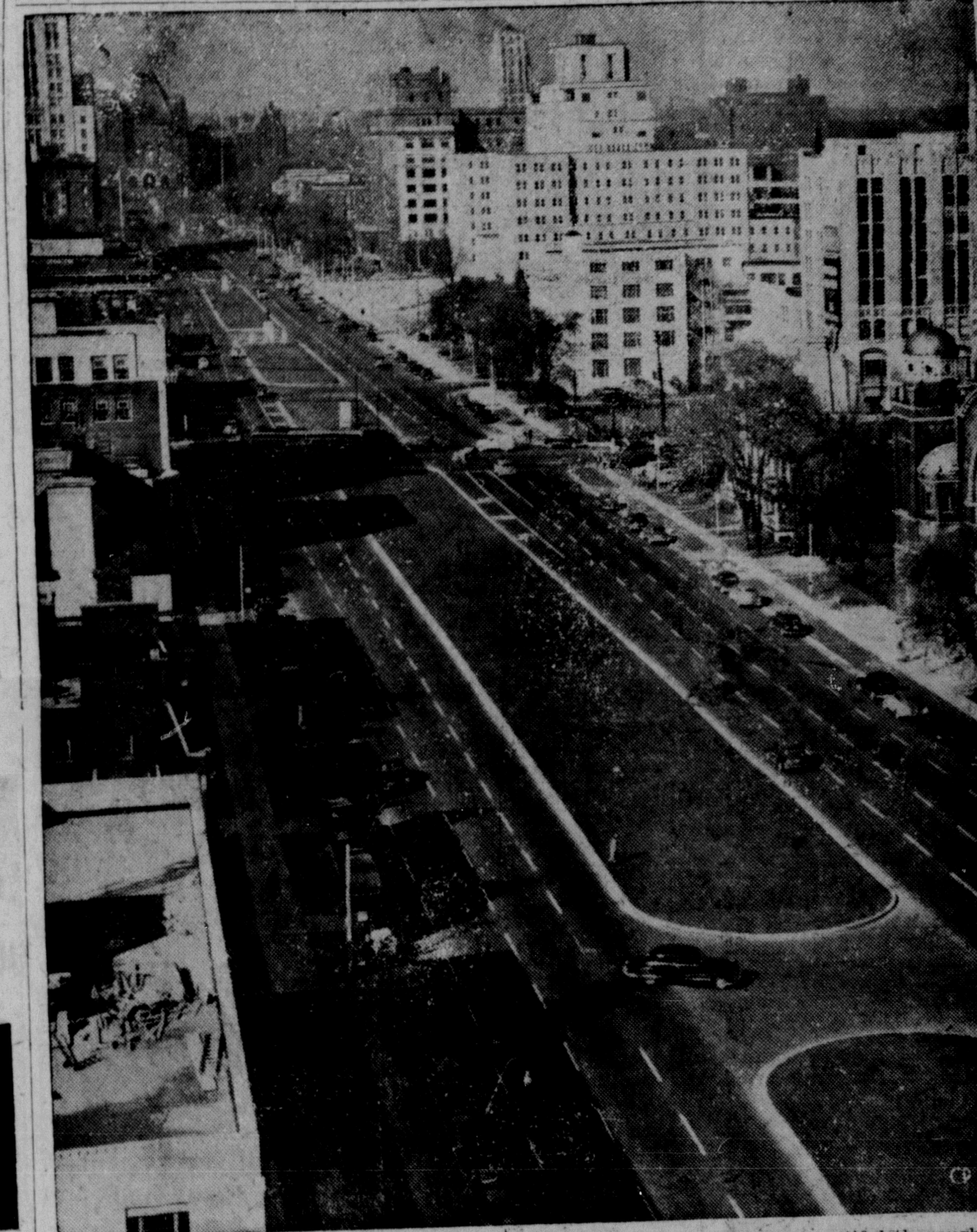
TO BEAUTIFY STREET—Here's University Avenue, one of Toronto's most beautiful thoroughfares. Those barren boulevards and the thin y-treed curbs will take on new beauty with the planting of small maple trees and shrubs. At lower left is the roof of the United States Consulate building; at top right, the new Hospital.
