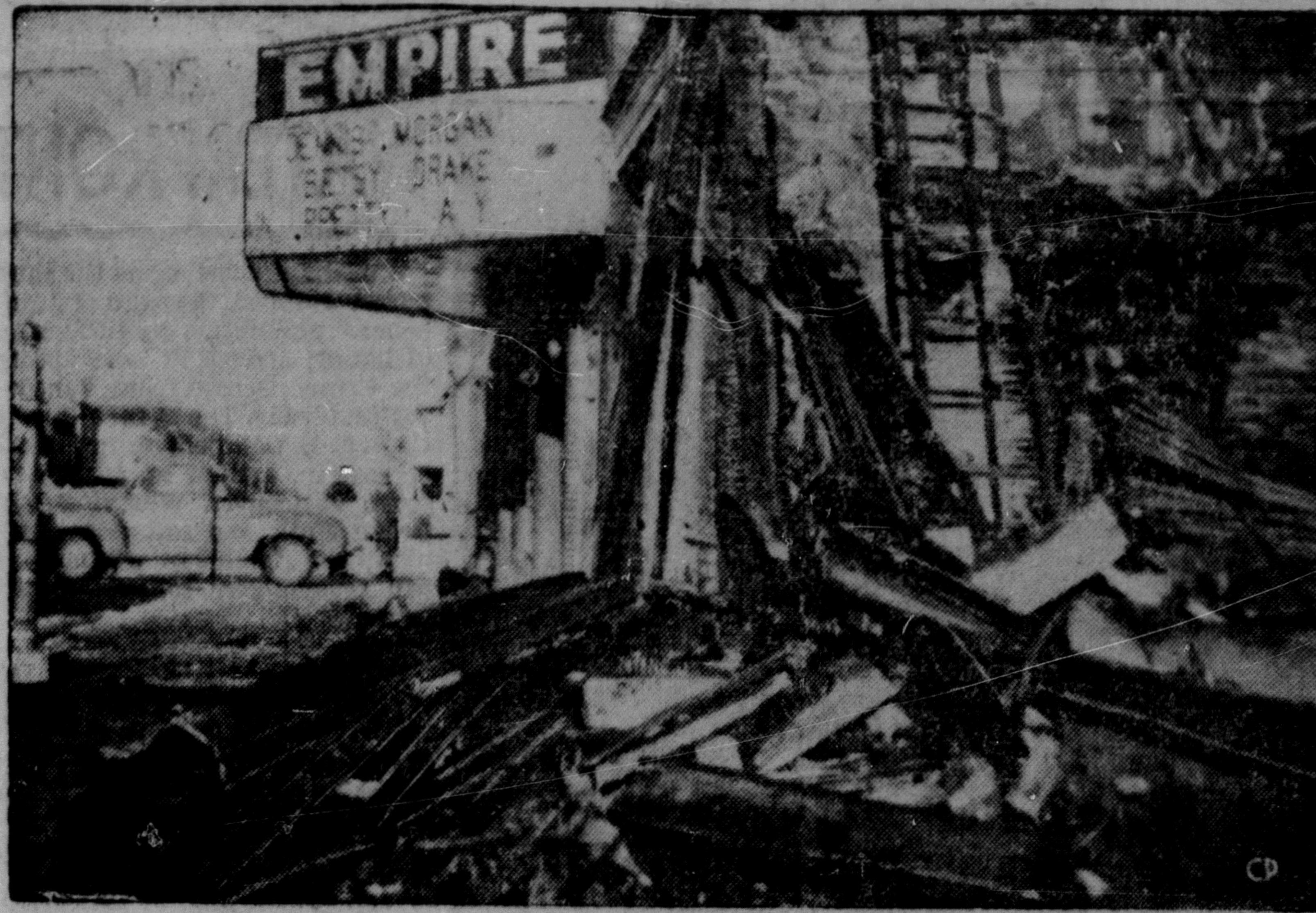
WALL SAVES THEATRE —Only a thick brick wall saved the Empire Theatre as flames engulfed four adjoining business blocks in a $500,000 fire in Thessalon, Ont. No one was injured, but 15 persons were made homeless. (CP PHOTO)
