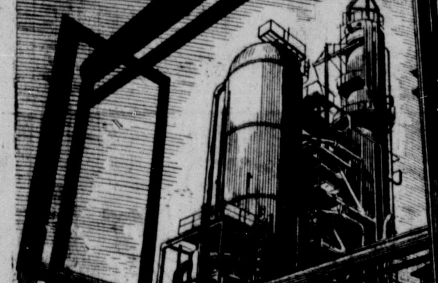
Much oil refinery equipment is made of Nickel alloys to stand up under intense heat, under subzero cold, and to resist corrosion by acids. The modern refinery contains hundreds of tons of Nickel alloys.
