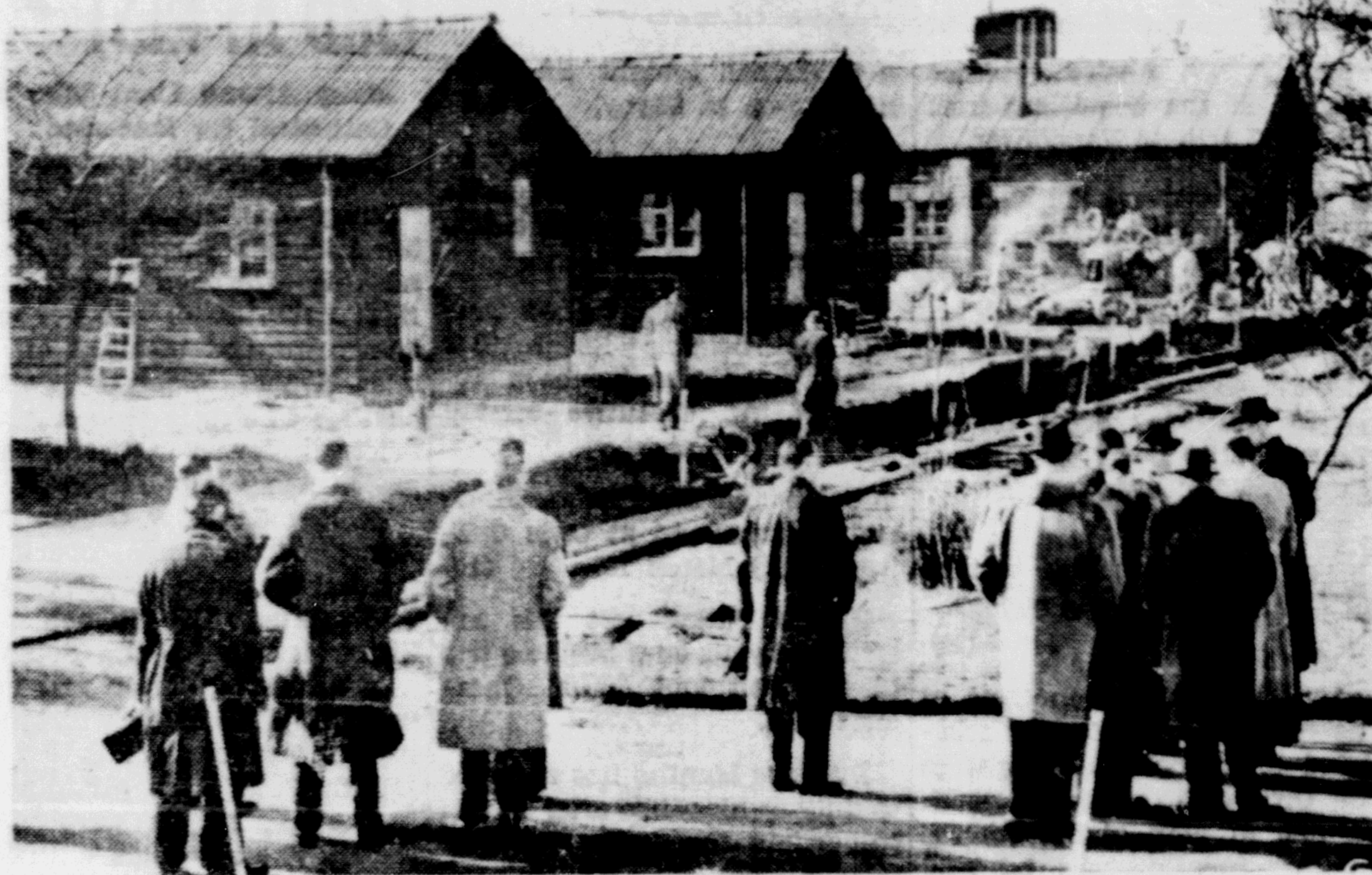
WHERE SUMMER OLYMPIC ATHLETES WILL LIVE IN LONDON—Here are some of the nearly completed houses in "Olympic Village" which is now under construction at Richmond Park, London, Eng., for the purpose of housing the members of the various international Olympic teams who will soon be arriving in England to participate in the forthcoming Olympic Games.
