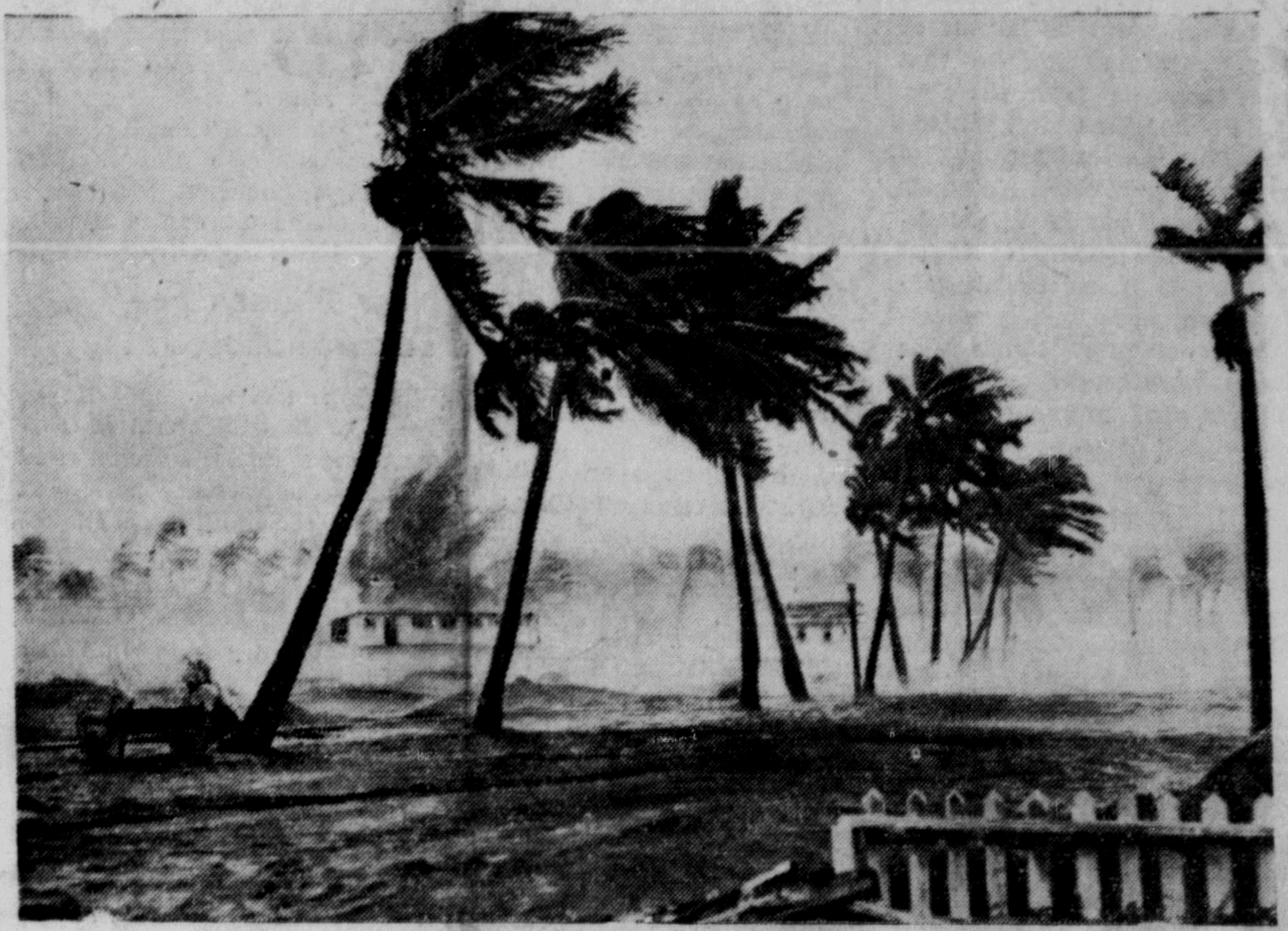
FLORIDANS TAKE TO CELLARS IN 150 M.P.H. HURRICANE—Bent over by the 150-mile-an-hour winds that lashed the Florida coast, this picture, taken at the height of the hurricane, shows one of the main thoroughfares in Palm Beach completely engulfed in water that was blown over the sea wall. Emergency shelters in many parts of the state were filled to capacity as the storm worked its way along the "Gold Coast," causing damage estimated in the millions.
