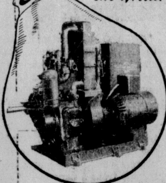
less to buy - and to operate than a gasoline plant; gives instant power and light, for as lew as 2c per K.W.H. . . . without storage batteries. Compact, yet fully equipped, the "switch-starting" machine is ready for use as soon as installed. The self-regulating "Morrison" generator, coupled direct to the Petter Diesel, runs at only 1,200 r.p.m. . . . continuously if required.
