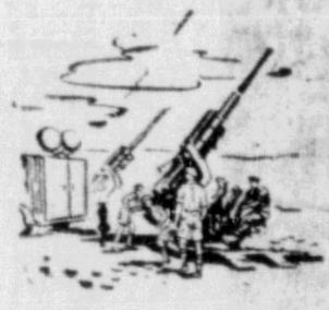
Science is playing an increasingly important role in Canada's new Army. In heavy anti-aircraft, for example, complex radar equipment predicts to within a few feet exactly where the target is and will be. The gunners, their backs to the target, fire with amazing accuracy by instrument.
