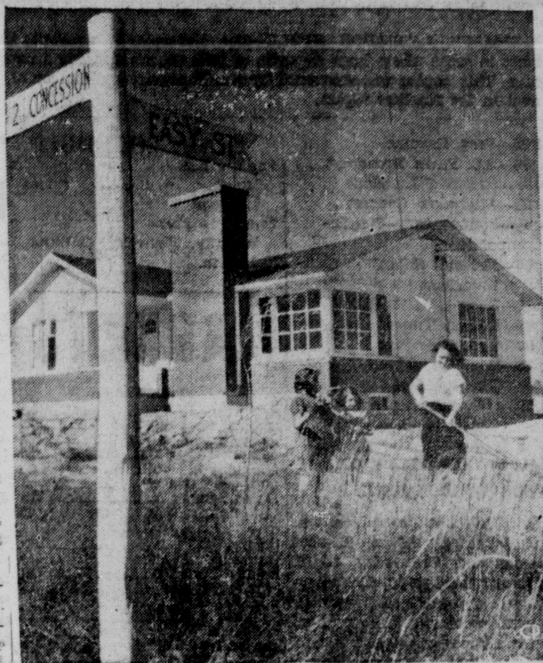
RIGHT ADDRESS —There is one family in London, Ont., living officially on Easy Street. Shown are Mrs. Floyd Osborne and her two young daughters landscaping their new home in a veterans' sub-division. The family was the first to build on an unnamed thoroughfare and the final result was so attractive, Mrs. Osborne named it Easy Street. (CP Photo)
