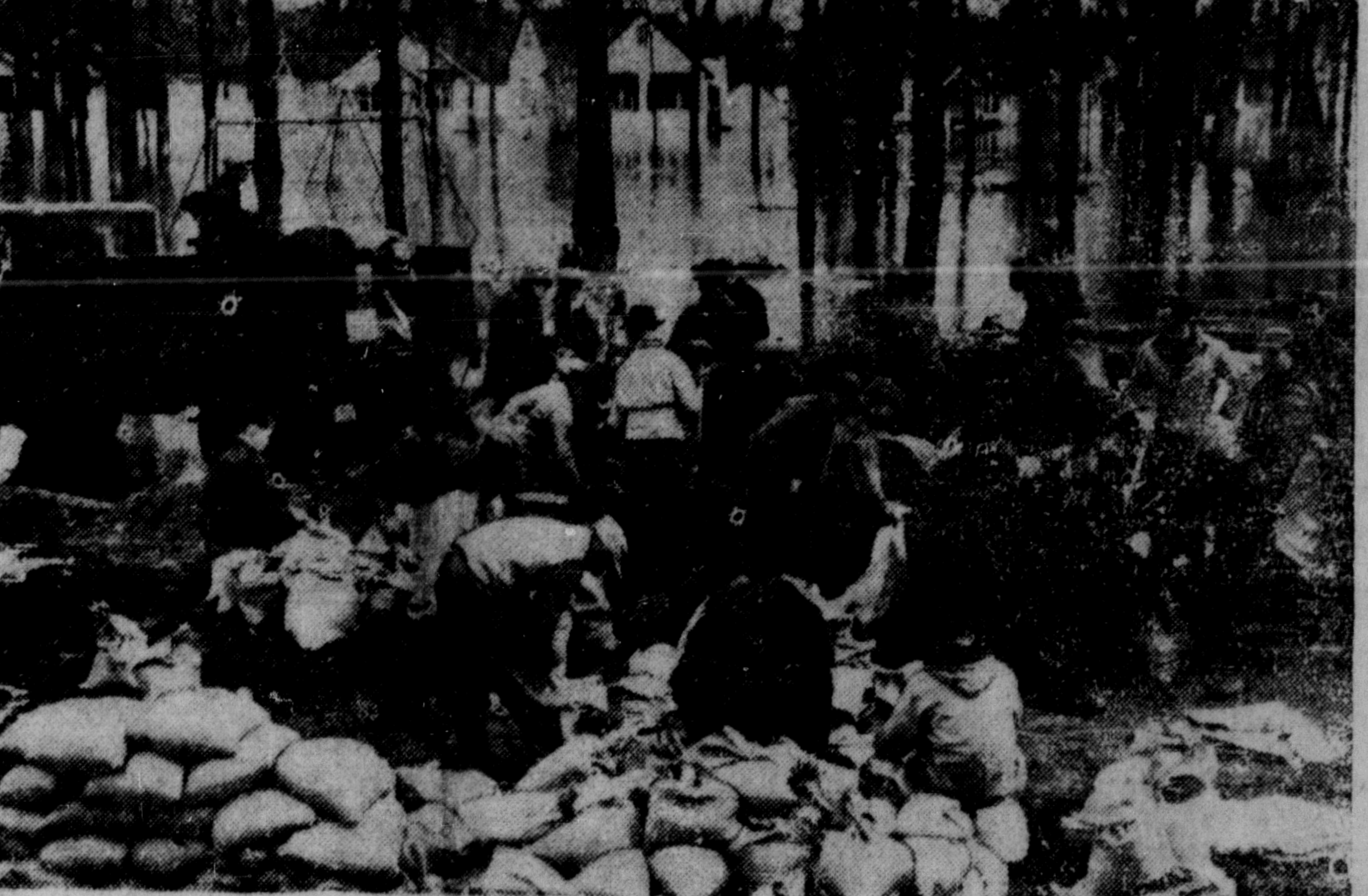
PARK BECOMES LAKE—Volunteer crews, part of a round-the-clock force, battle the rising Red River at Elm Park in St. Vital a Winnipeg suburb. Hundreds of sandbags are being thrown up to keep the river from the valuable residential property. On the left is an army truck used in helping fight the floods. (CP Photo)
