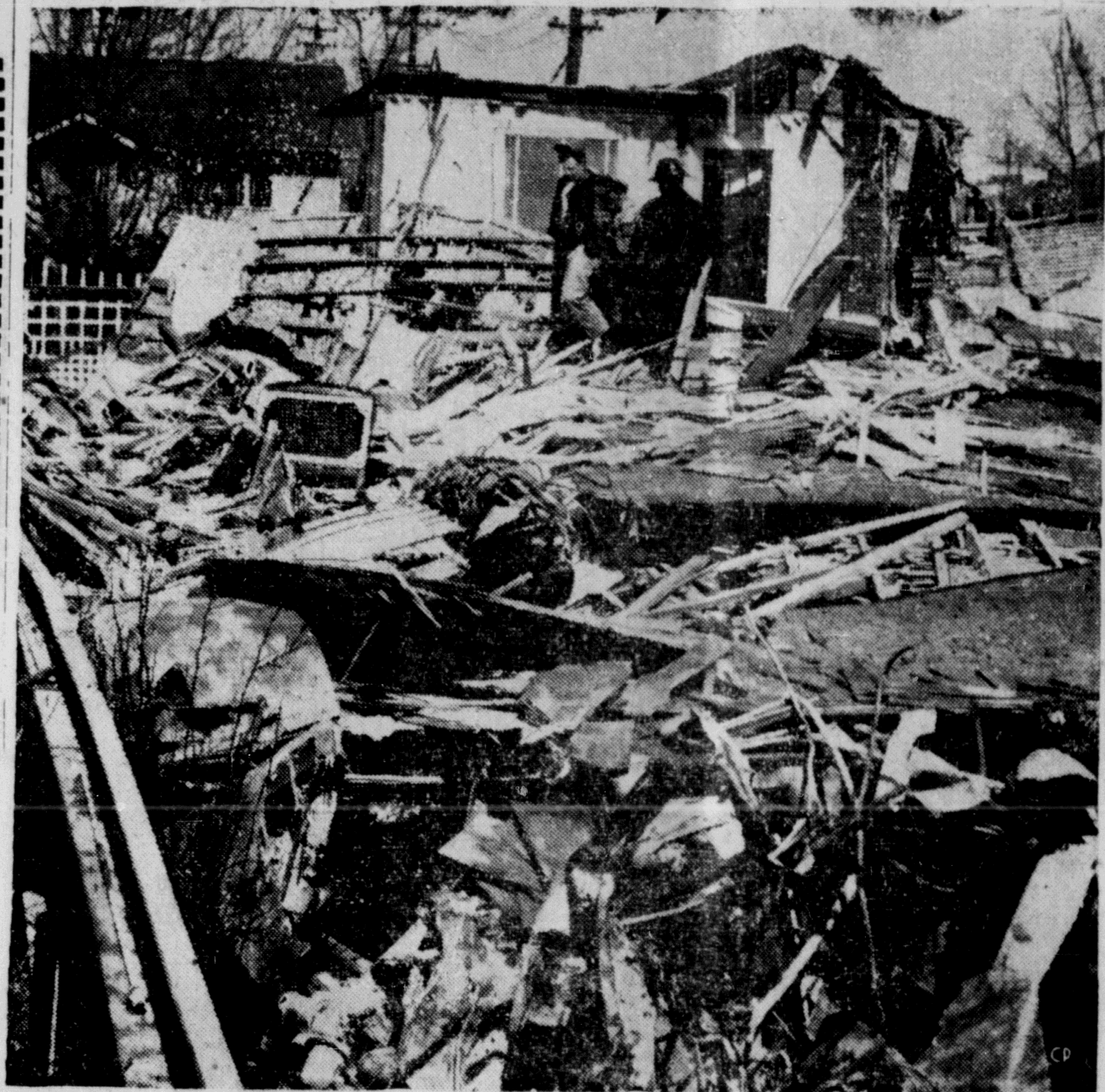
NARROW ESCAPE —The four occupants of this house escaped severe injury when the five-room bungalow on Calgary's North Hill was demolished in a plane crash. Jack Harper, 22-year-old pilot of the twin-engine Cessna, was instantly killed. Police said they were told by witnesses that Harper, a salesman for an aviation company, had been drinking before he took one of his company's planes on the night-time rooftop-hopping flight. Shown in the background centre is the last remaining wall of the house of Marshall McDougall, a police station switchboard operator. The debris in the foreground includes both the plane and the house. (CP Photo)
