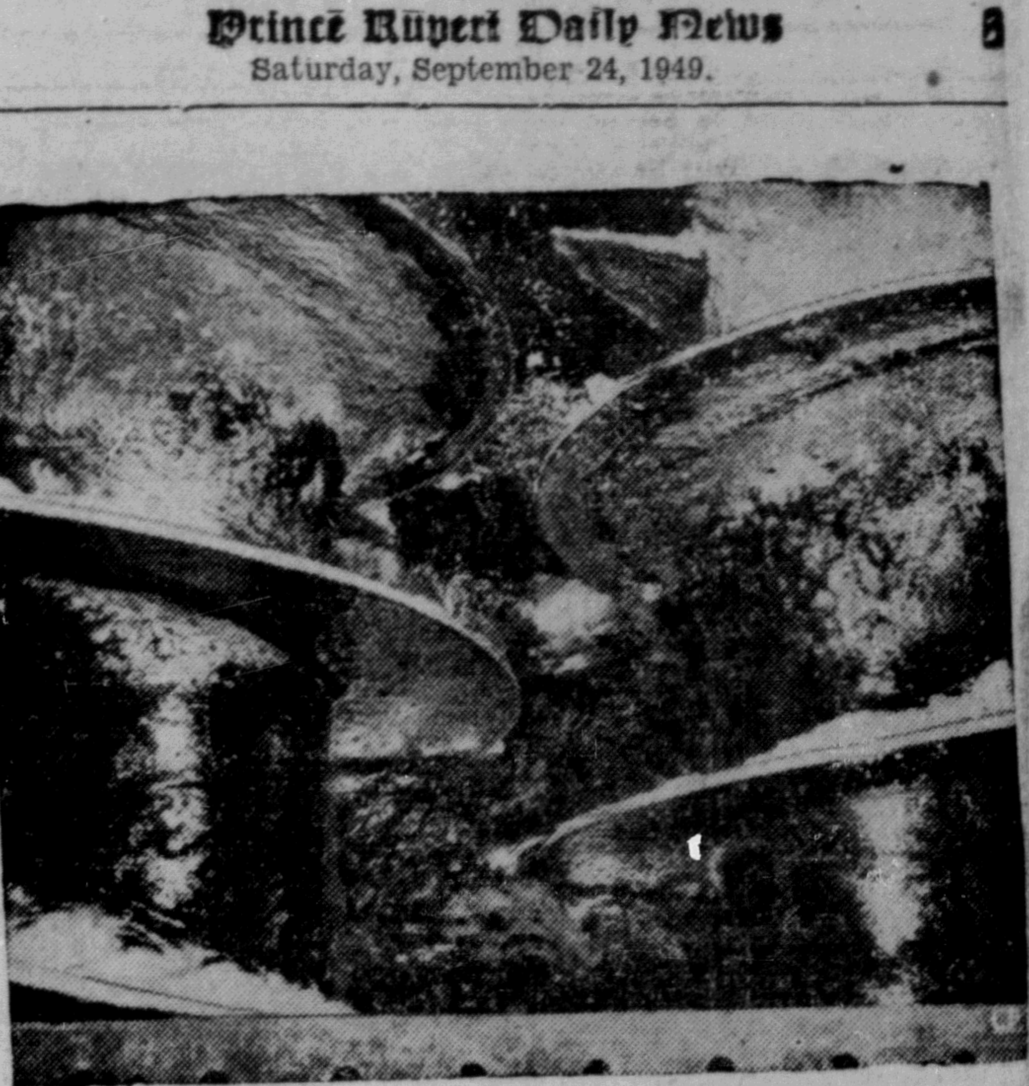
DRIPPING SAND —Steamed and mixed with hot water, the rich Northern Alberta tar sand is processed for oil at the Alberta Government's experimental plant at Bitumont. Here the mixture is churned at the top of a conveyor belt carrying it through the plant which has produced an average of 250 barrels of oil daily this summer. (C. P. Photo)
