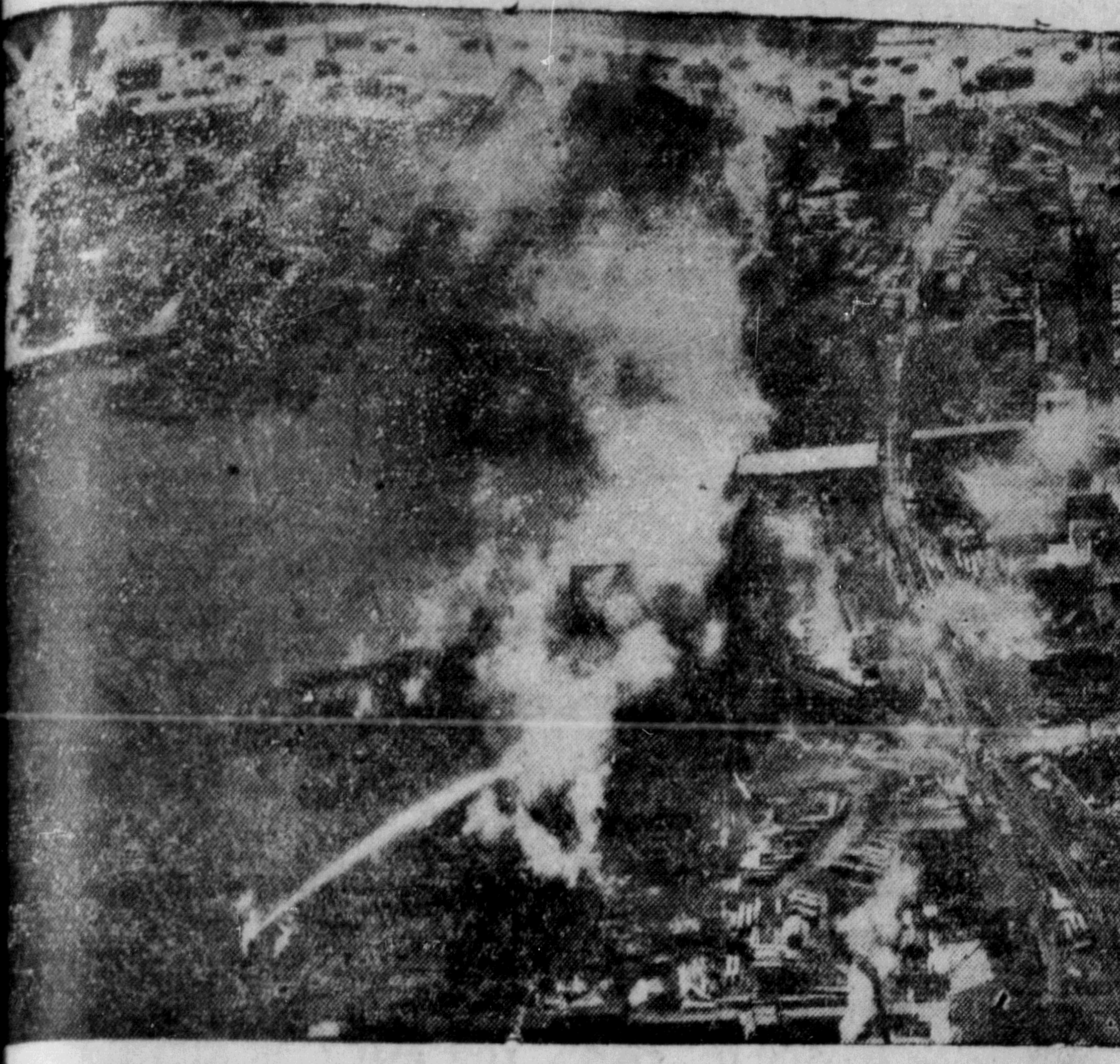
FIRE —Vancouver's industrial False Creek area still smoldered 6½ hours after the blaze that swept three blocks of factories and injured 13 persons. This aerial view shows the fireboat J. H. Carlisle pouring water on the embers of the fire, which razed and destroyed 13 buildings. (C. P. Photo)
