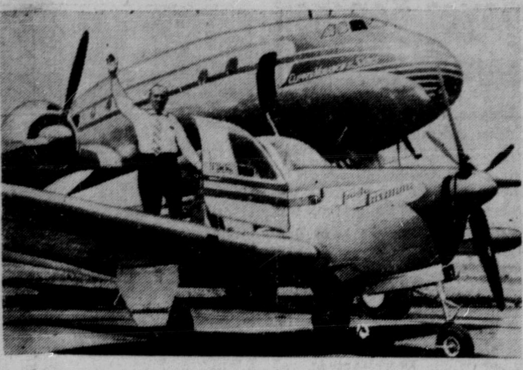
TO TRY EAST-WEST LINDBERGH-John Brondello, 36, Italian engineer, waves from the single-engine plane in which he hopes to make the first east-west single-engine plane crossing of Atlantic, accompanied by co-pilot. This photo was taken before plane was dismantled and flown to London aboard DC-4. Extra fuel tanks and navigation aids have been installed for the hop which will start at Lisbon, Portugal.
