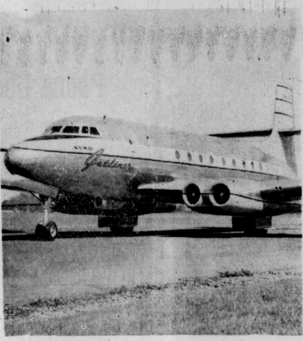
CONTINENT'S FIRST JET AIRLINER-Canada's jet airliner, the only jet passenger plane in the western hemisphere, has passed its test flight at Malton Airport, Ont. Four-engined the plane will fly at 400 m.p.h. at 30,000 feet. It climbed 12,000 feet, flew 250 m.p.h. in its first trial.
