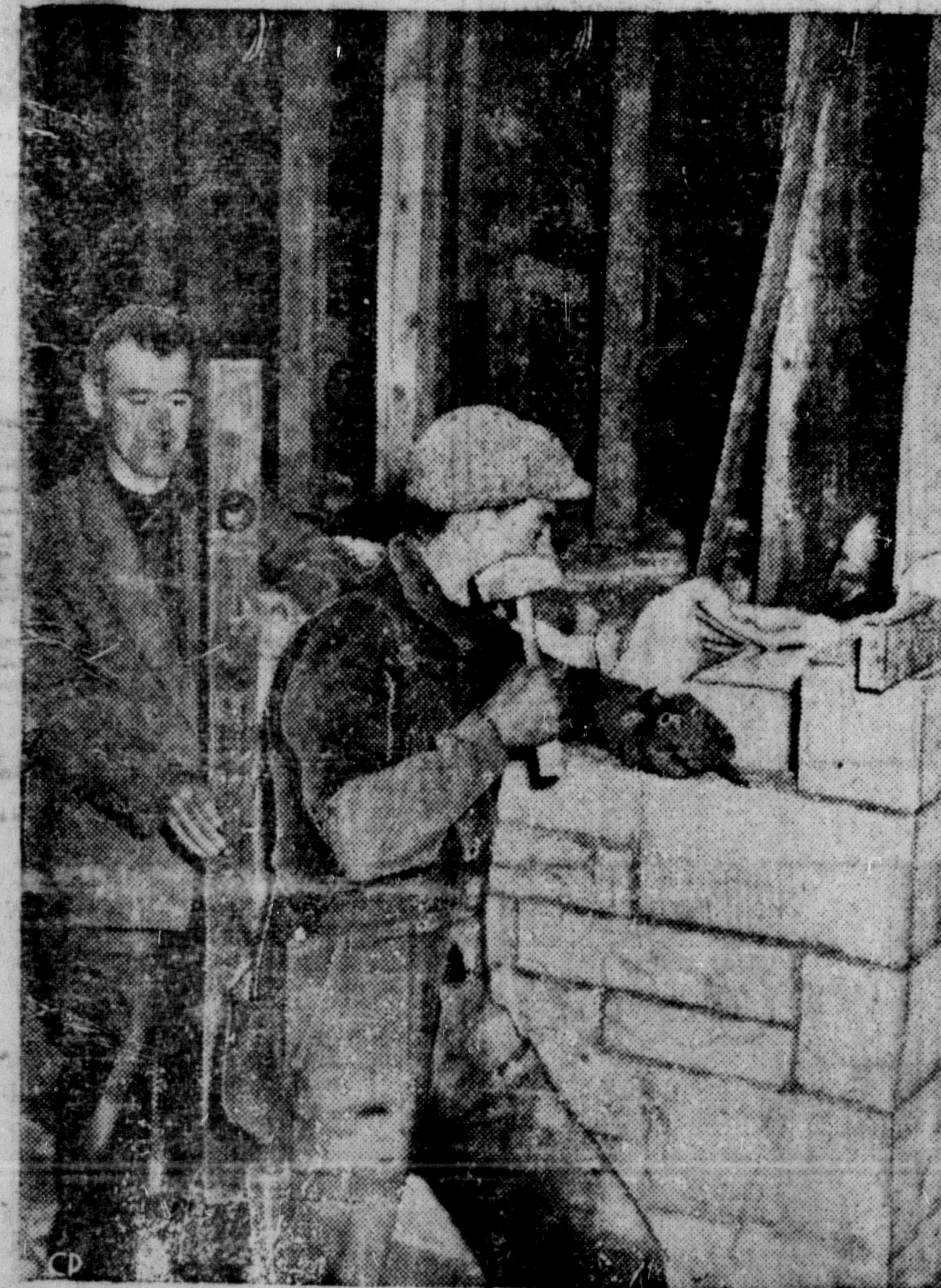
FLYING BUILDERS —Stonemasons are so scarce in Canada that four were flown from Scotland to London, Ont., to speed up the building of Thames Hall, University of Western Ontario athletic building. Builders say there are less than 100 of the artisans in Canada. At work, left to right, are George King, Sid Hird and Norman Murray. (CP Photo)
