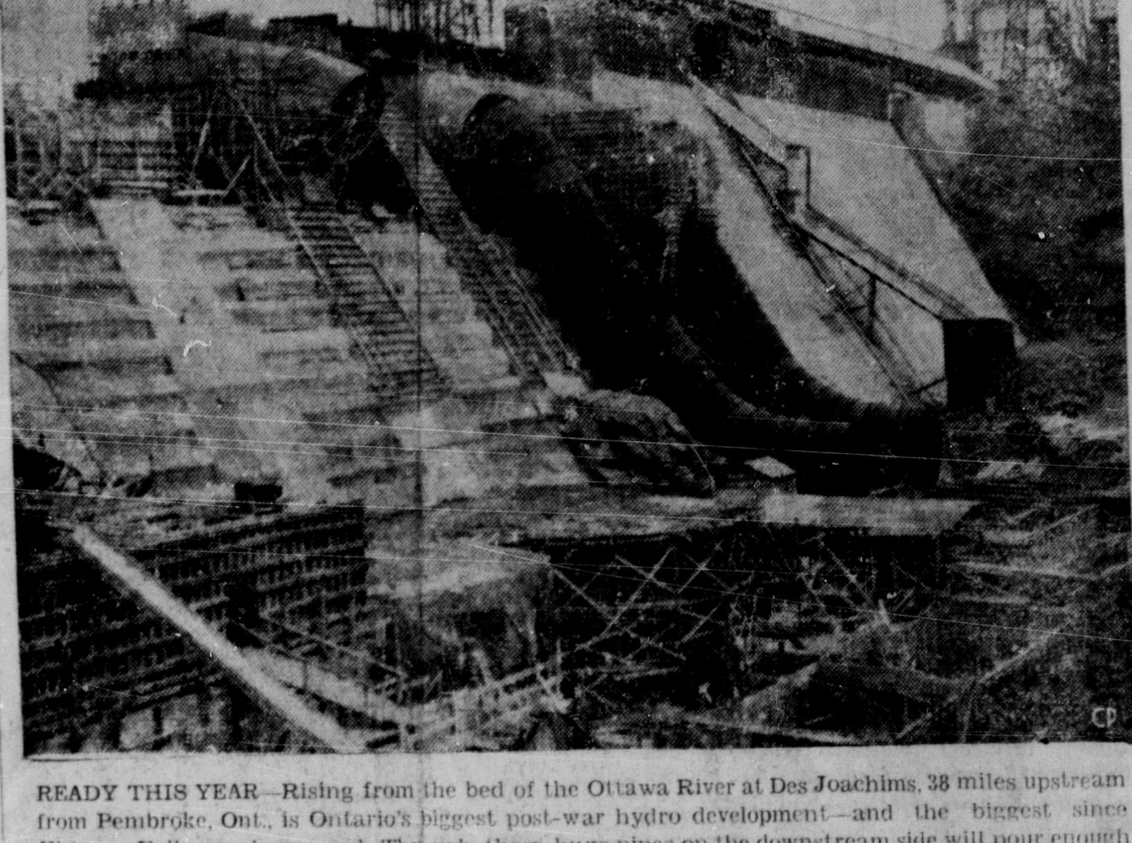
from Pembroke, Ont., is Ontario's biggest post-war hydro development-and the biggest since Niagara Falls was harnessed. Through these huge pipes on the downstream side will pour enough water to generate almost 480,000 horsepower of electrical energy. Some 2,500 men have worked for three years on the Des Joachims project; its first units are scheduled to go into operation in
