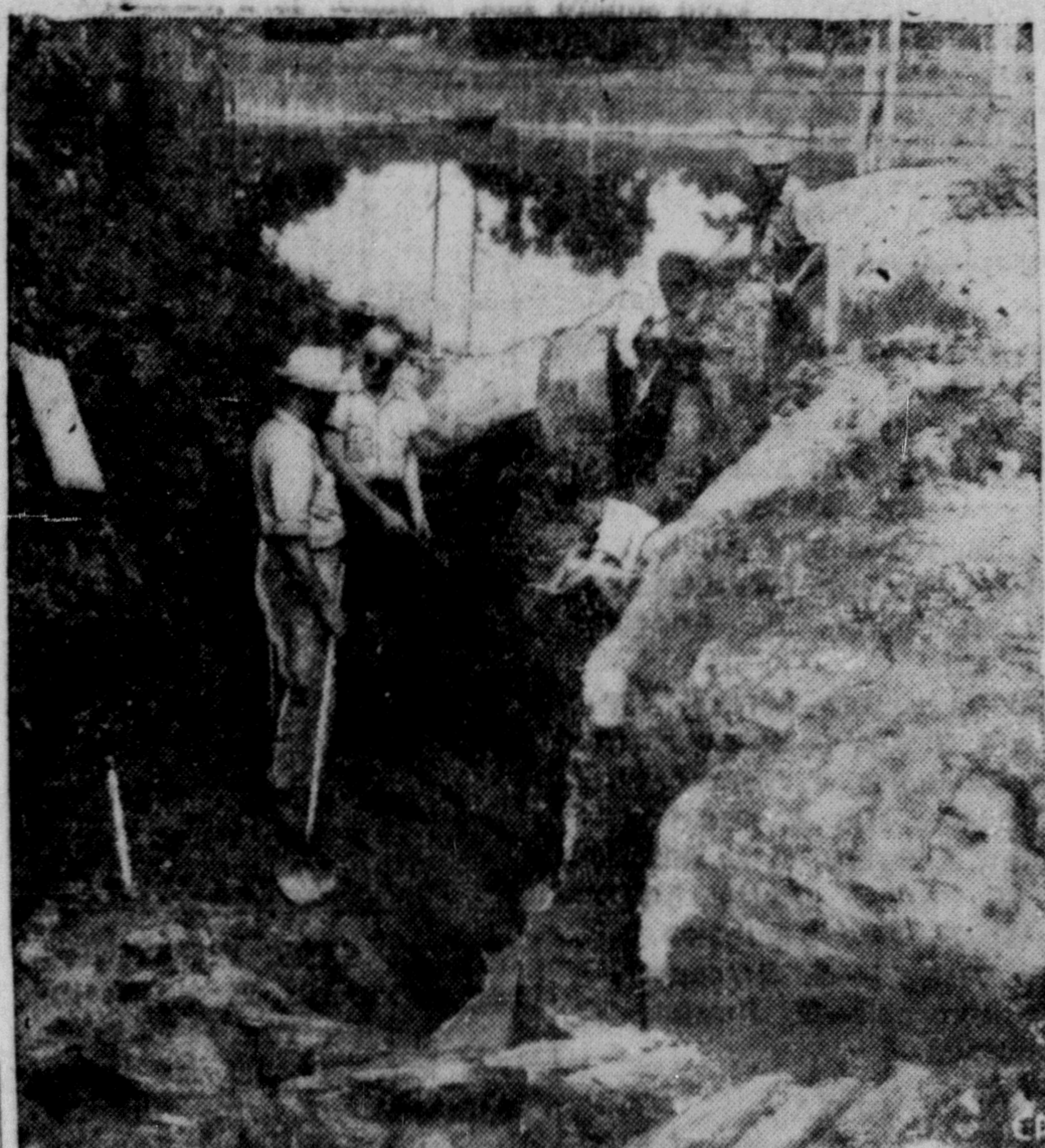
FIRST CANAL—The first known canal lock system in North America has been uncovered in excavations at the old Huron fort of Ste. Marie, near Midland, Ont. Wilfred A. Jury, curator of the University of Western Ontario, who directed the investigations, stands beside the timber sides of the old canal, burned to ground level when the Hurons abandoned the Jesuit stronghold to the Iroquois 300 years ago. (C. P. Photo)
