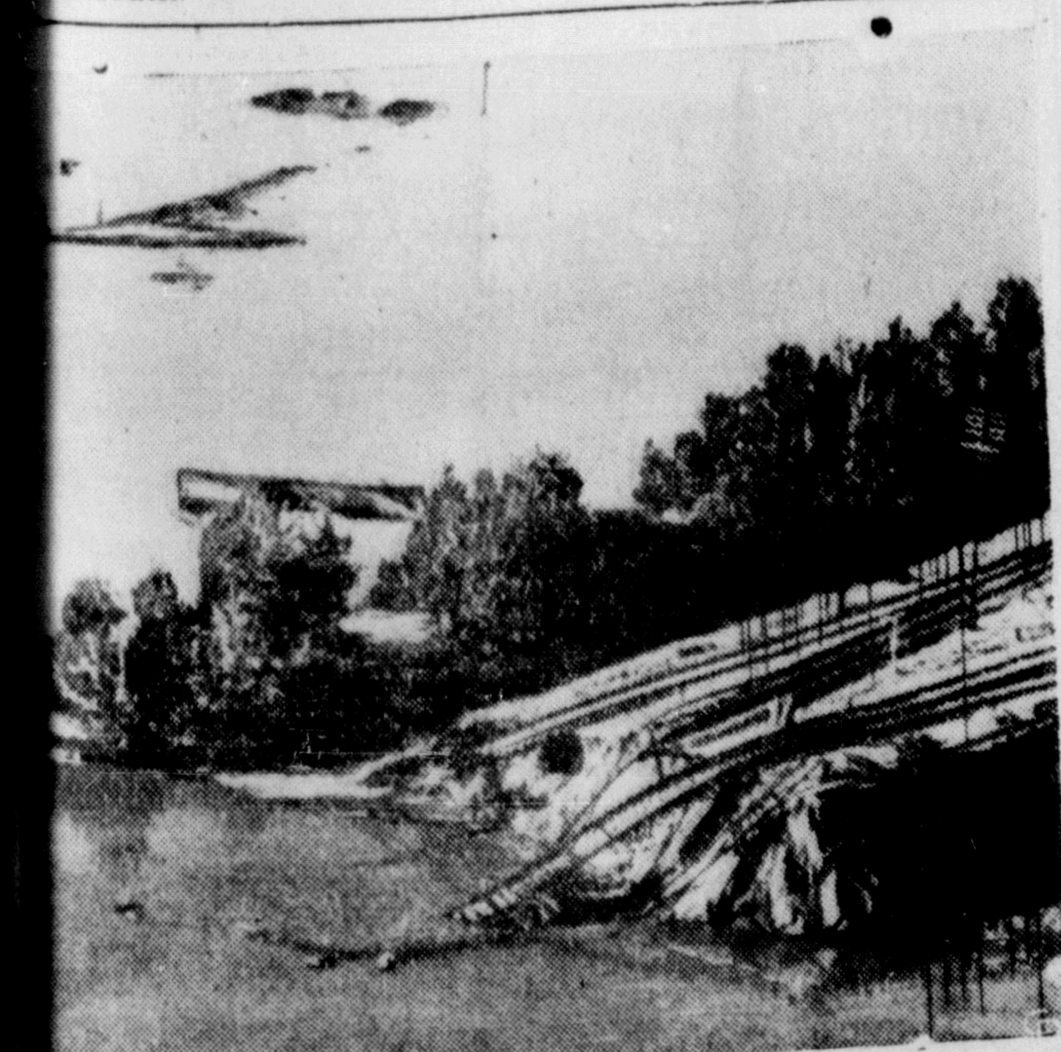
DISASTER POURS INTO VANPORT—Railroad tracks trail off the embankment which was pierced by Columbia River, allowing flood waters to swamp Vanport, Oregon. The war-built city, 3,700 residents was completely destroyed. The railroad fill, built about 40 years ago, had previously been checked and declared strong enough to withstand the flood.
