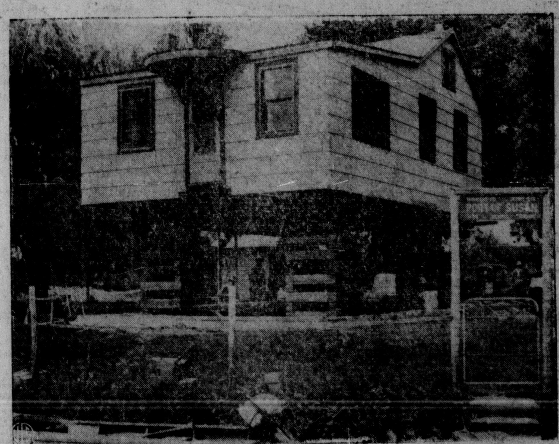
HIGH LIFE—This cottage on Frentress Lake in Dubuque, Iowa, is getting a "high rise." The uplifting, accomplished by wooden blocks, will bring the dwelling out of the reach of flood waters in case the Mississippi River rises to flood level again. The area is on a "cut-off" from the river and was flooded in 1951 and 1952.
