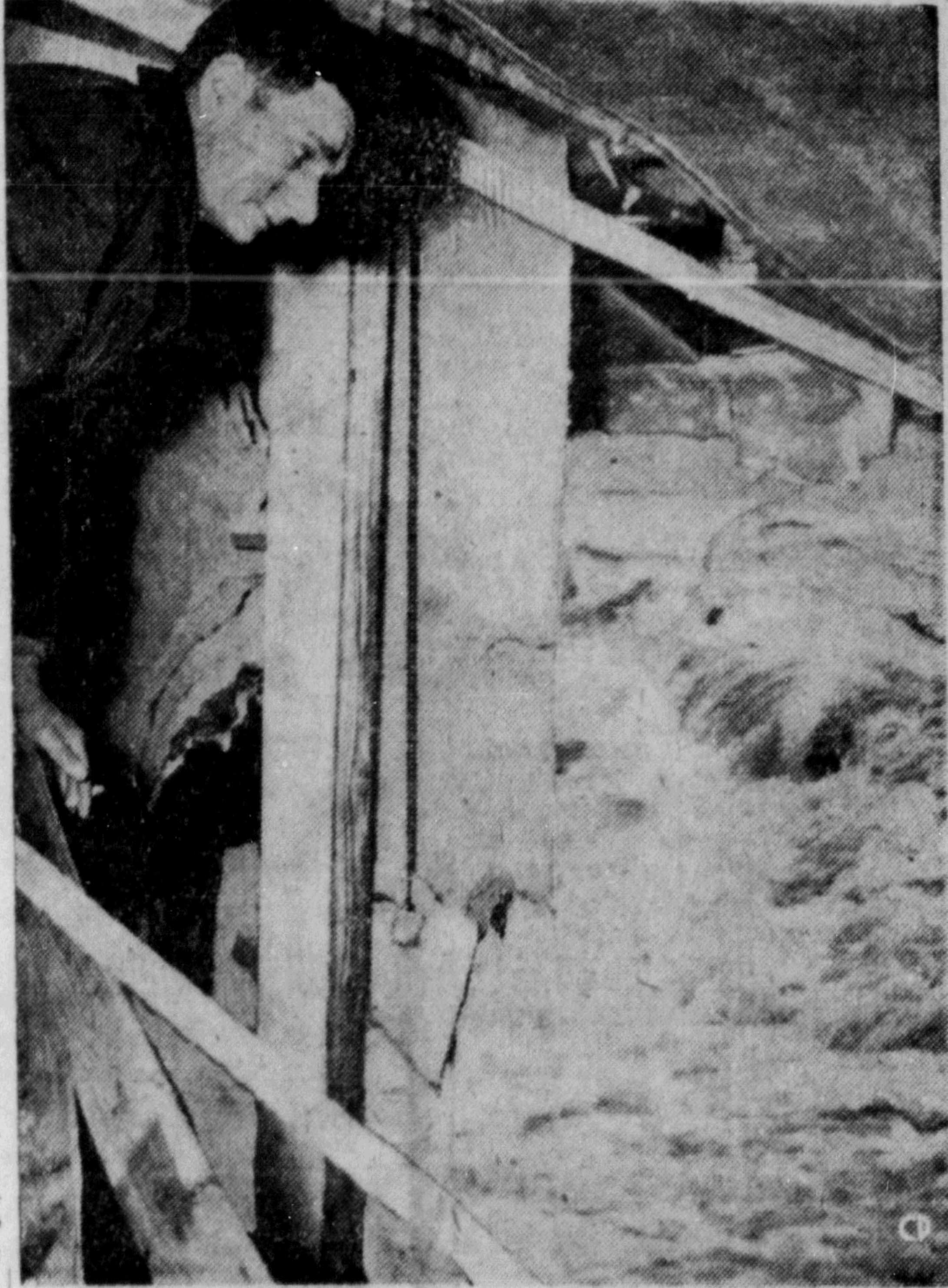
GALE WRECKS HOUSE—George Cairns of Toronto's suburban Long Branch looks sorrowfully at the raging waters of Lake Ontario which have torn away the living room and two bedrooms and flooded the remainder of his home. In Long Branch 44 families were left homeless and 21 houses were condemned as unfit for human habitation in on-the-spot checks by village councillors. The storm extended all along the Great Lakes area from Oshawa to Windsor and damage was heavy. (CP Photo)
