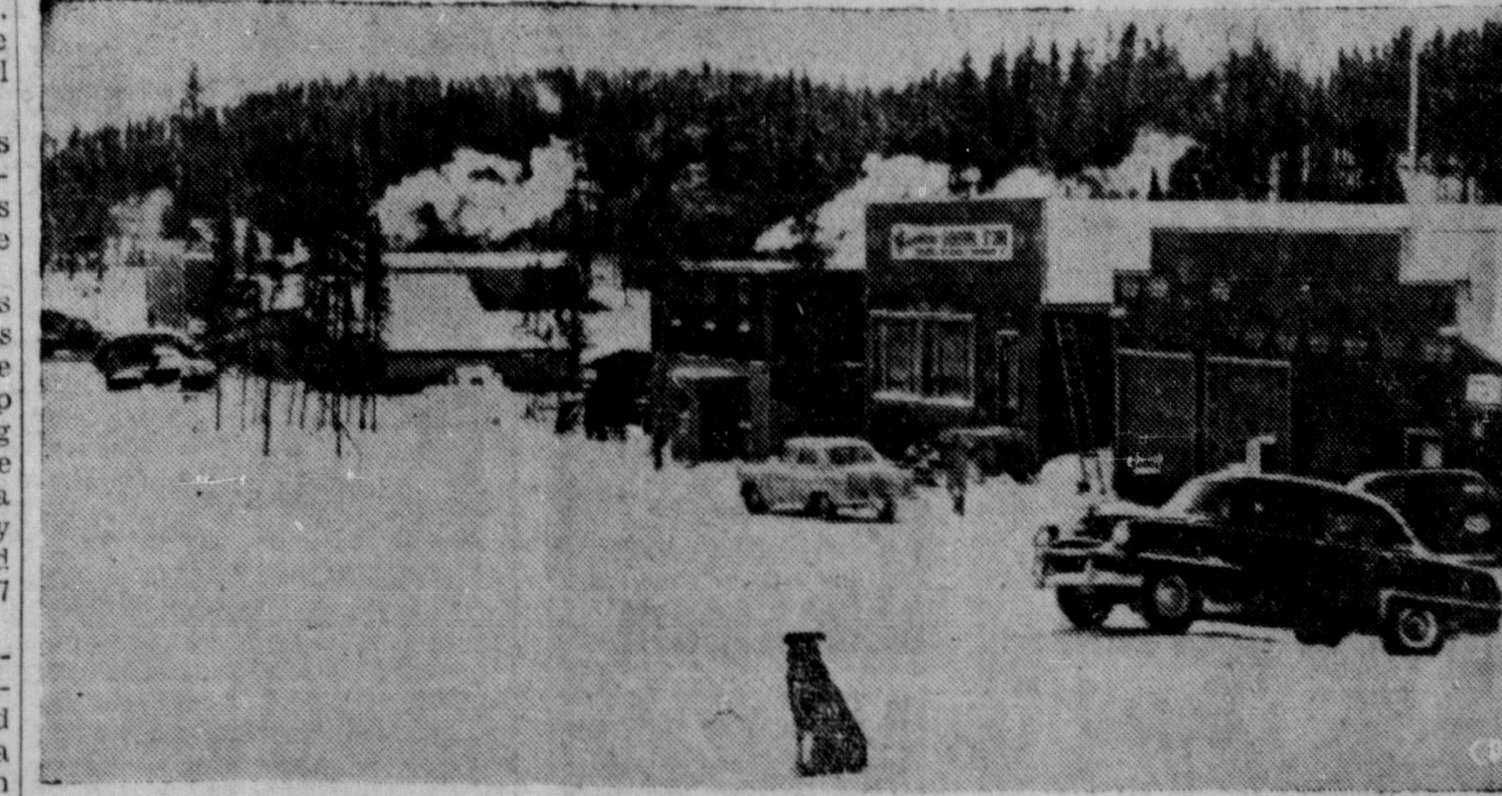
THE MINING COMMUNITY OF URANIUM CITY in northern Saskatchewan has shown remarkable progress since the provincial department of natural resources began carving the townsite out of the wilderness in June, 1952. When the hunt for uranium started, incoming prospectors threw up haphazard rows of flimsy shack-tents and one-room shanties. These have been replaced by well-planned business sections and modern homes and schools. Pictured is part of Uranium road showing garages, taxi stand, general store, lumber yard.
