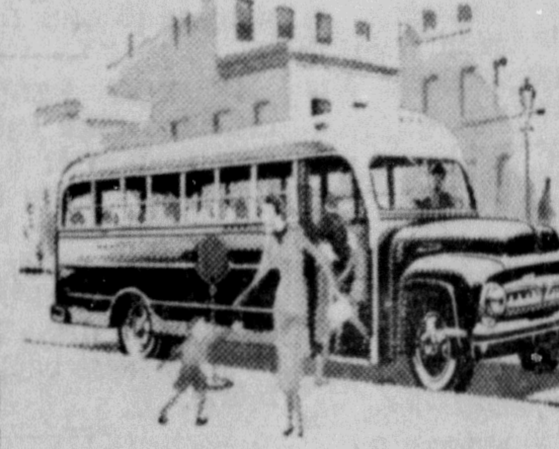
2 School Bus Series—F-600 (illustrated)—G.V.W. 15,000 lbs. for up to 54 passengers. Also F-750—G.V.W. 20,000 lbs. for up to 66 passengers.
