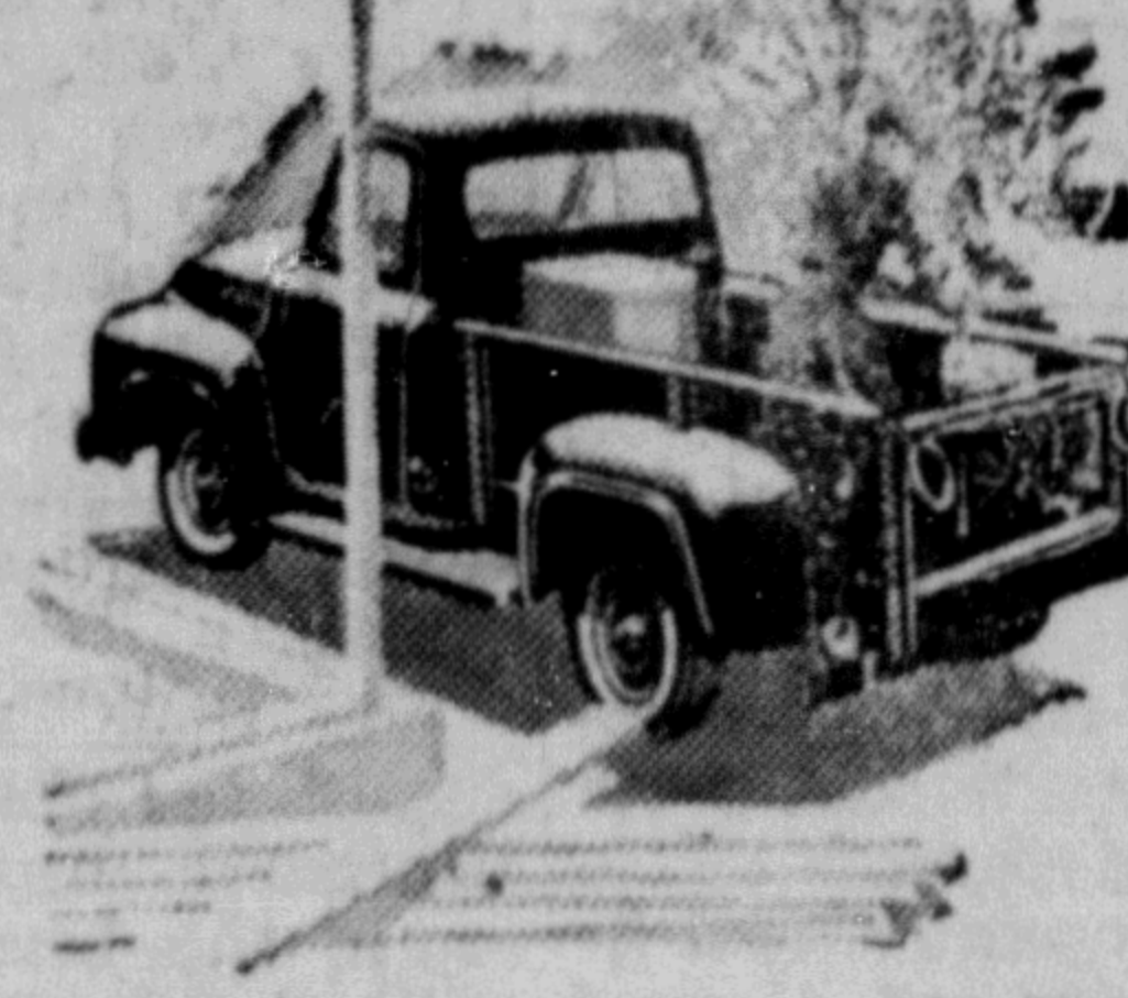
F-250 8-ft. Express—G.V.W. 6,900 lbs. Payload up to 3,107 lbs. New bolted body construction.
