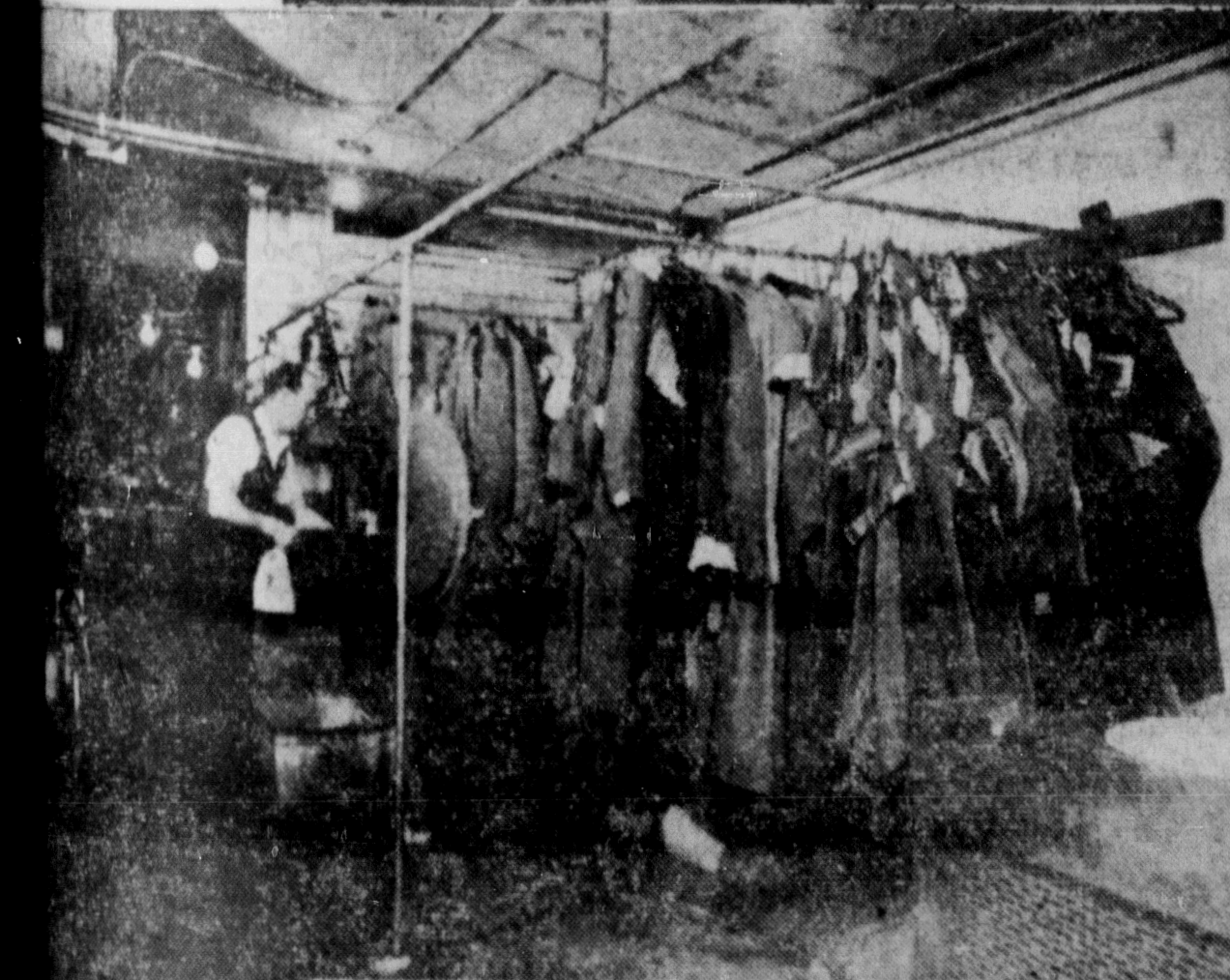
This room is located next to the dry cleaning room. The machine in the back, showing the operator in front of it, is the deodorizing machine in which all dry cleaning fumes are eliminated by way of fresh, clean, heated air. It also shows racks with dry-cleaning hanging up ready for the steam spotting process.
