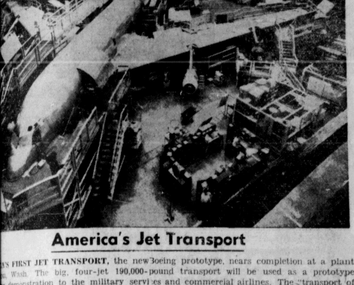
TRANSPORT, the new3oeing prototype, nears completion at a plant wash. The big, four-jet 190,000-pound transport will be used as a prototype demonstration to the military services and commercial airlines. The "transport of re" is 128 feet long and its wings measure 130 feet from tip to tip. The cruising speed 550-m.p.h. class. The military version will be used as a multi-purpose, tanker-transa commercial airliner, the giant will be capable of regular transcontinental non-stop
