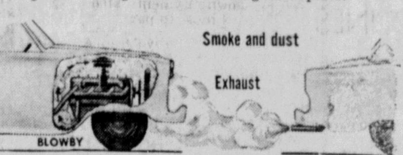
Then Standard scientists discovered the real cause: Exhaust vapors and crankcase fumes contain tiny bits of soot, gum and dust. They're drawn in with the air your engine needs and stick in the carburetor.
