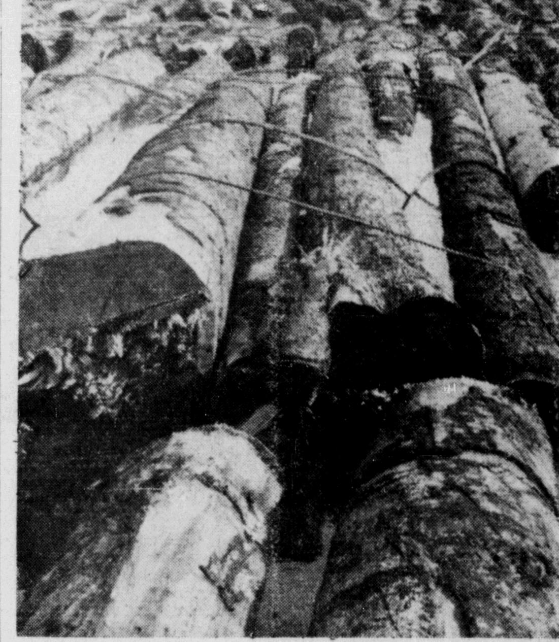
BUNDLE RAFT"-First such experiment of towing huge amount of logs over great distances-is composed of bundles of logs interlaced with heavy "weaving cable." Raft landed at Columbia Cellulose Co. pulp mill last week. This system will be used by the company for all future towing.
