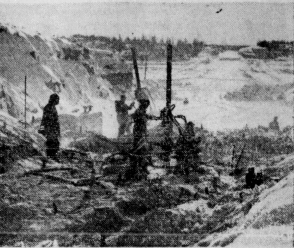
Despite snow and sub-zero temperature, construction work continues on the highways of Northern Ontario. Drillers are busy on a 15-foot cut on Highway No. 17 between Sudbury and Whitefish. Completed drill holes are plugged to keep out water until ada. In a deep, insidious sort of Historically, dairy men have dynamite can be inserted. The project involves removing thousands of tons of rock and hauling hundreds of thousands
