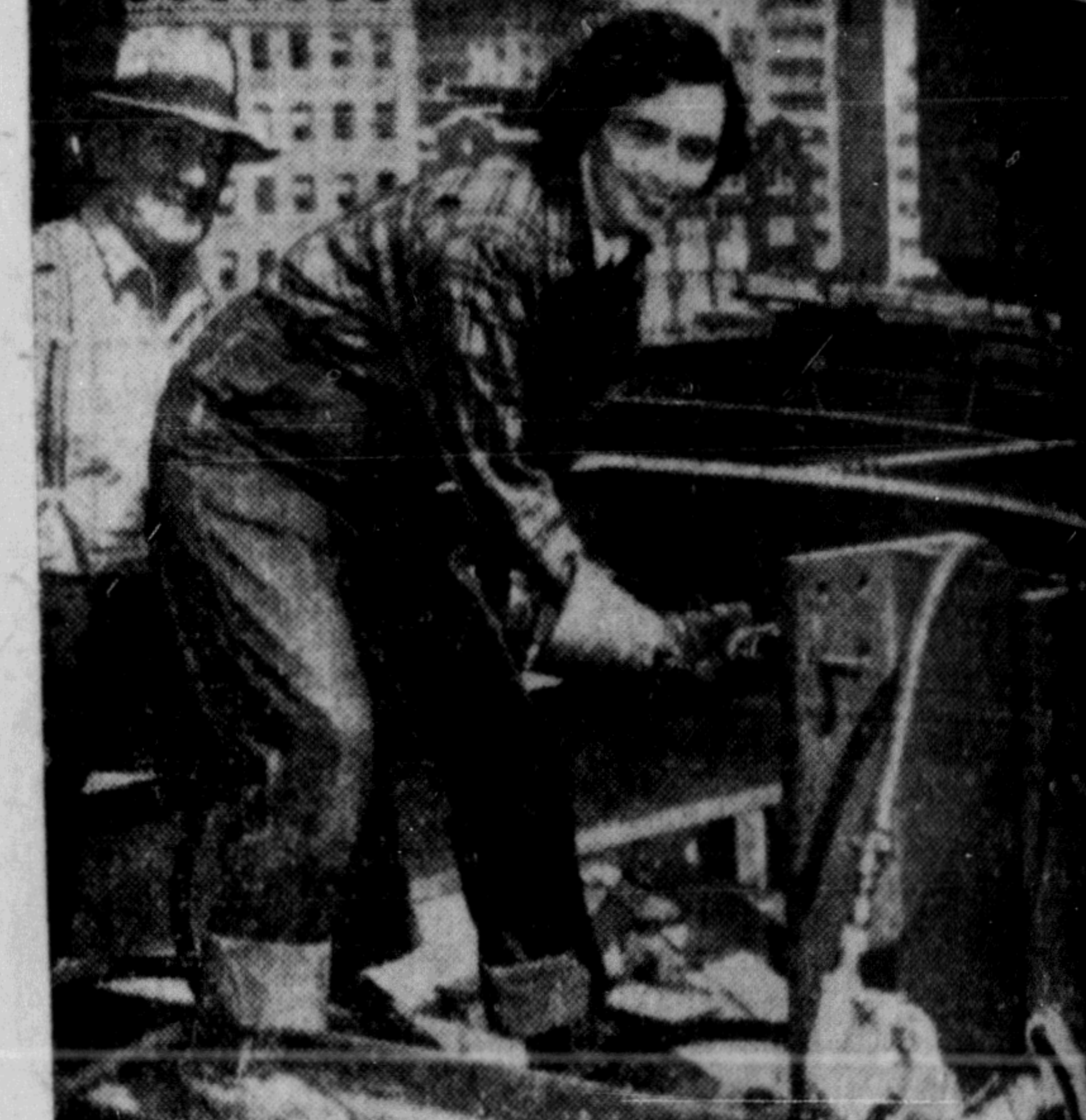
CAROL TARLTON, third-year engineering student, is getting some practical experience during vacation from McGill University. Here, she is six storeys up on a building under construction in downtown Montreal trying her skill at a rivet. Foreman George Lerfrance gives her a helping hand.
