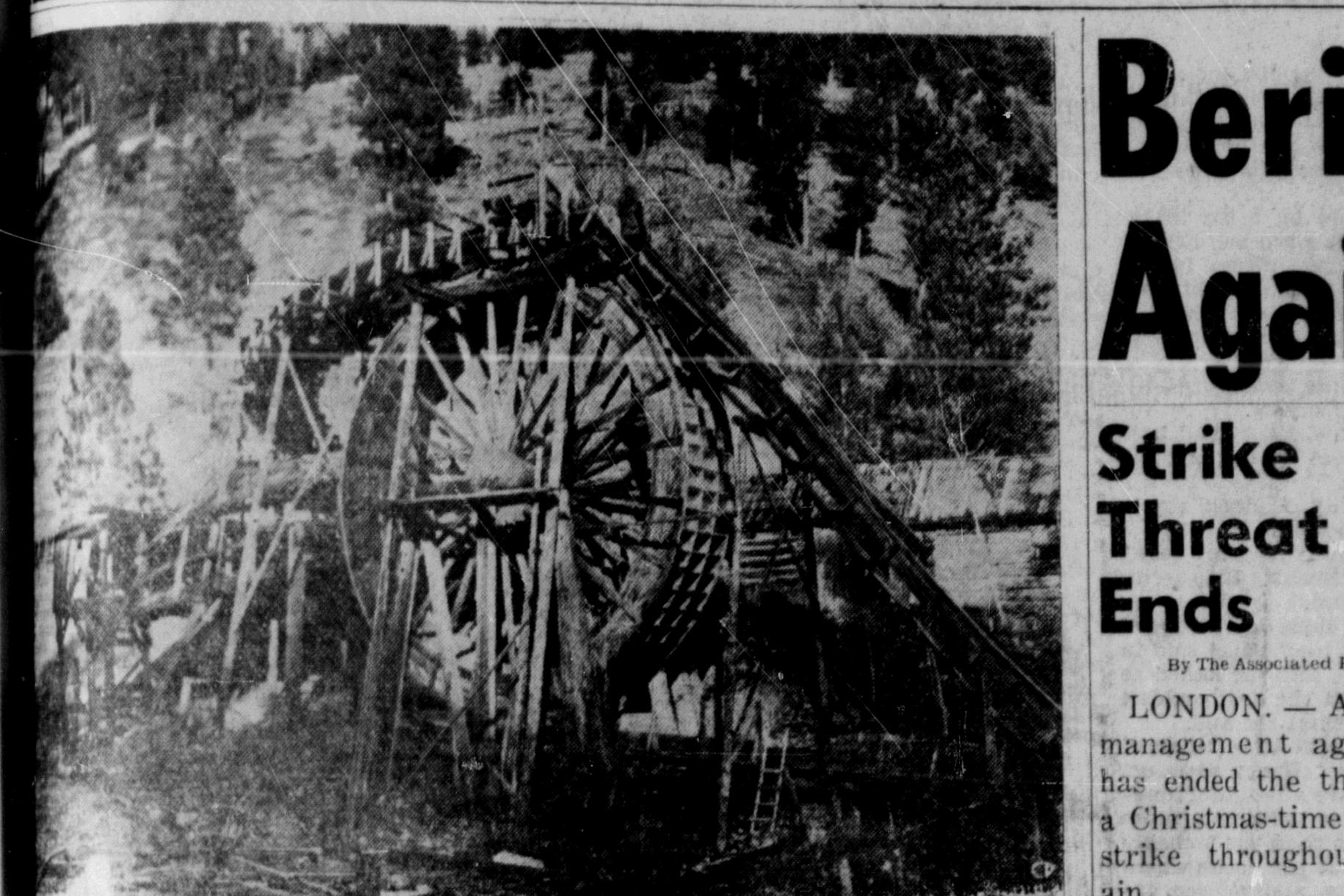
TRIS WATER WHEEL, so big it looks like a ferris wheel, was erected on Perry Creek, 15 miles north of Cranbrook, B.C., in 1933 when placer miners were crowding Perry Creek for gold. Built from 11,000 board feet of lumber it powers two pumps used to drain seepage from a mine 100 feet deep. When built the wheel was considered the largest of its kind in North America. It is 32 feet in diameter, has a seven-foot face width and 72 built-in-buckets.
