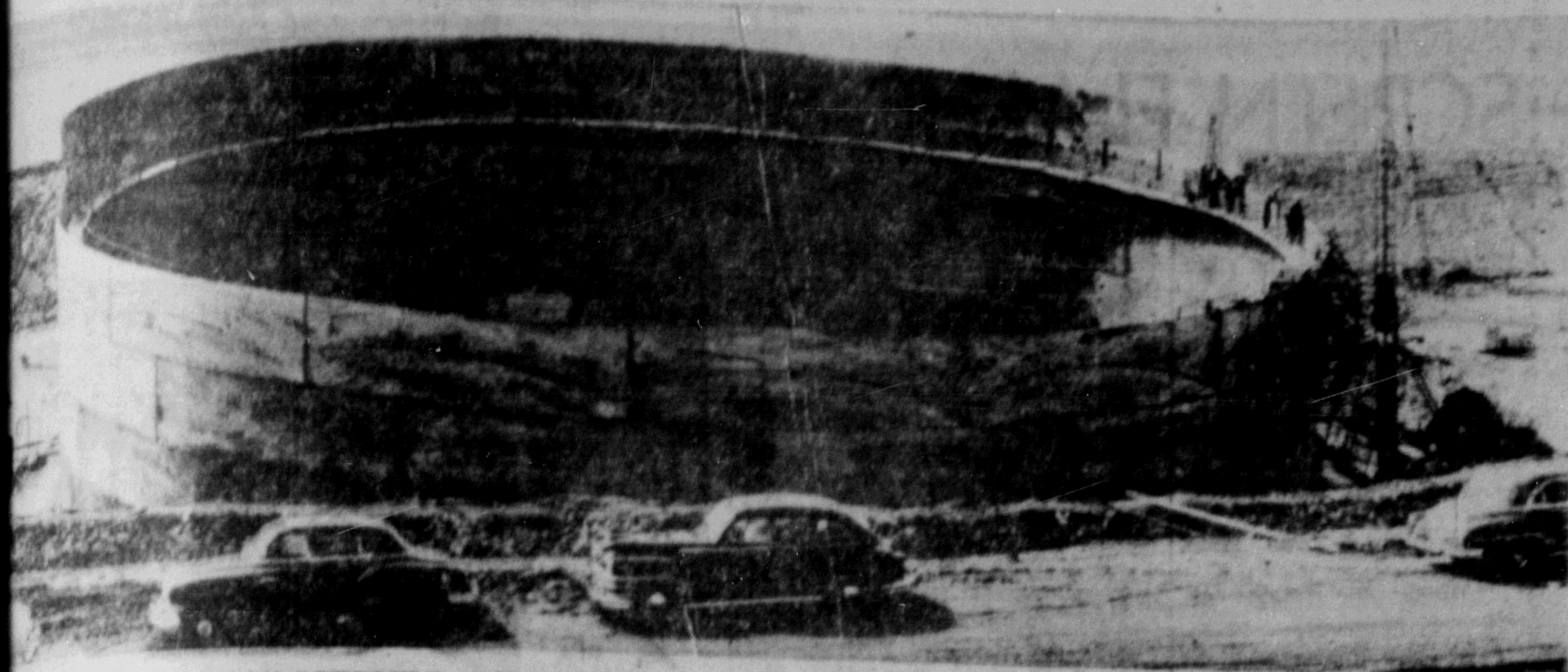
IS PROGRESSING ON SCHEDULE at Trans Mountain Line Company crude oil tank farm at Burnaby. This shows construction of the first 150,000-barrel tank. The
