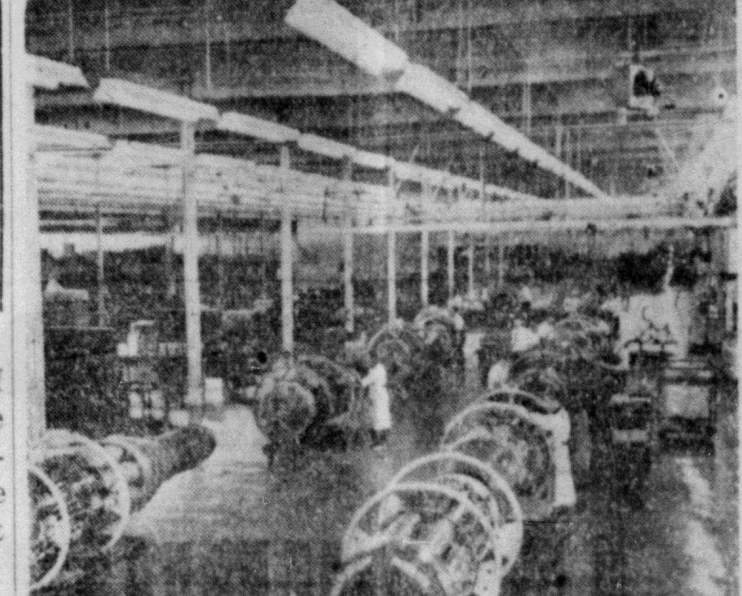
THIS IS THE PRODUCTION LINE where Sabre jet engines are overhauled at a new plant near Toronto's suburban Downsview airport. The plant was built and staffed by Canadian General Electric Campany under an arrangement with the defence departmana
