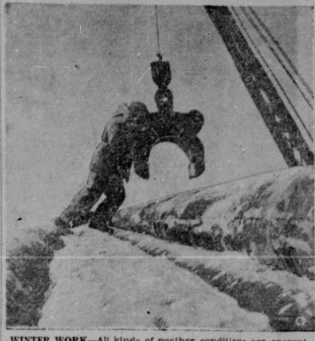
WINTER WORK-All kinds of weather conditions are encountered in the laying of the pipelines which are forming a steel tube from the Great Lakes to Vancouver for the transportation of Western Canada's oil. Heavy pipe lengths are handled by of a three-year contract at a mechanical tongs guided by warmly-clad workmen. (CP PHOTO)
