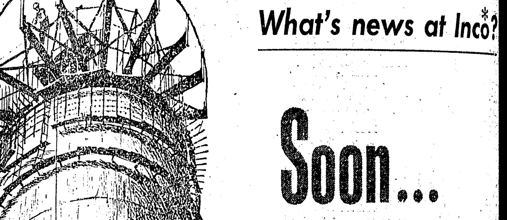
615 feet above some high ground near Copper Cliff, Ontario, the tallest chimney in the British Commonwealth will soon rear its nickel-chrome stainless steel crown.
