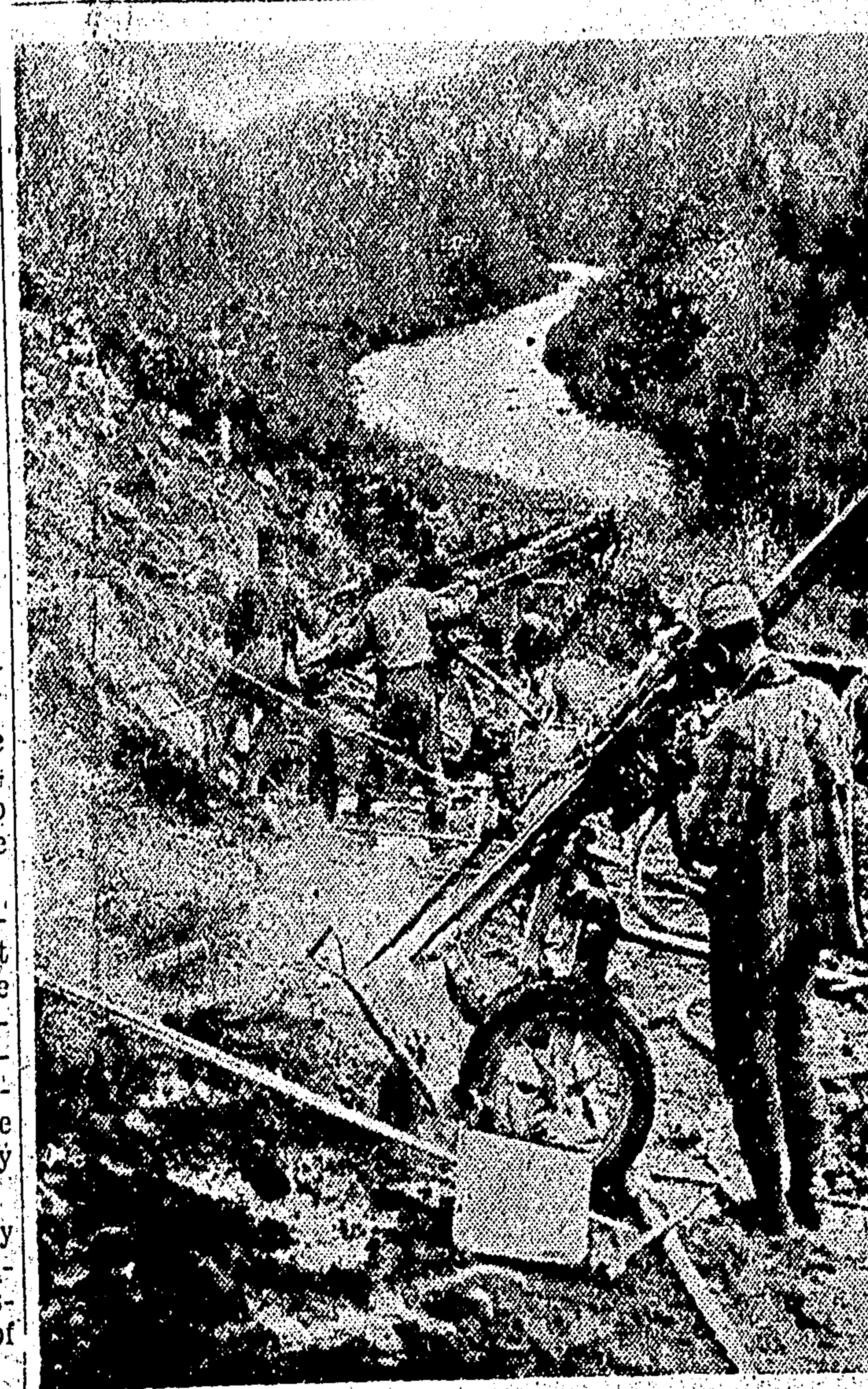
DRILLERS PREPARE HOLES to be filled with dynamite that will blast a giant section of sidehill in the Cran River valley near St. Felicien, Quebec, where Canadian National Railways is building a frontier railroad into the Chibougamau mining district. The 200-mile railway will swing from Beatyville through the Chibougamau district, which is approximately 400 air miles north of Montreal, then to Lake St. John. (CP Photo).
