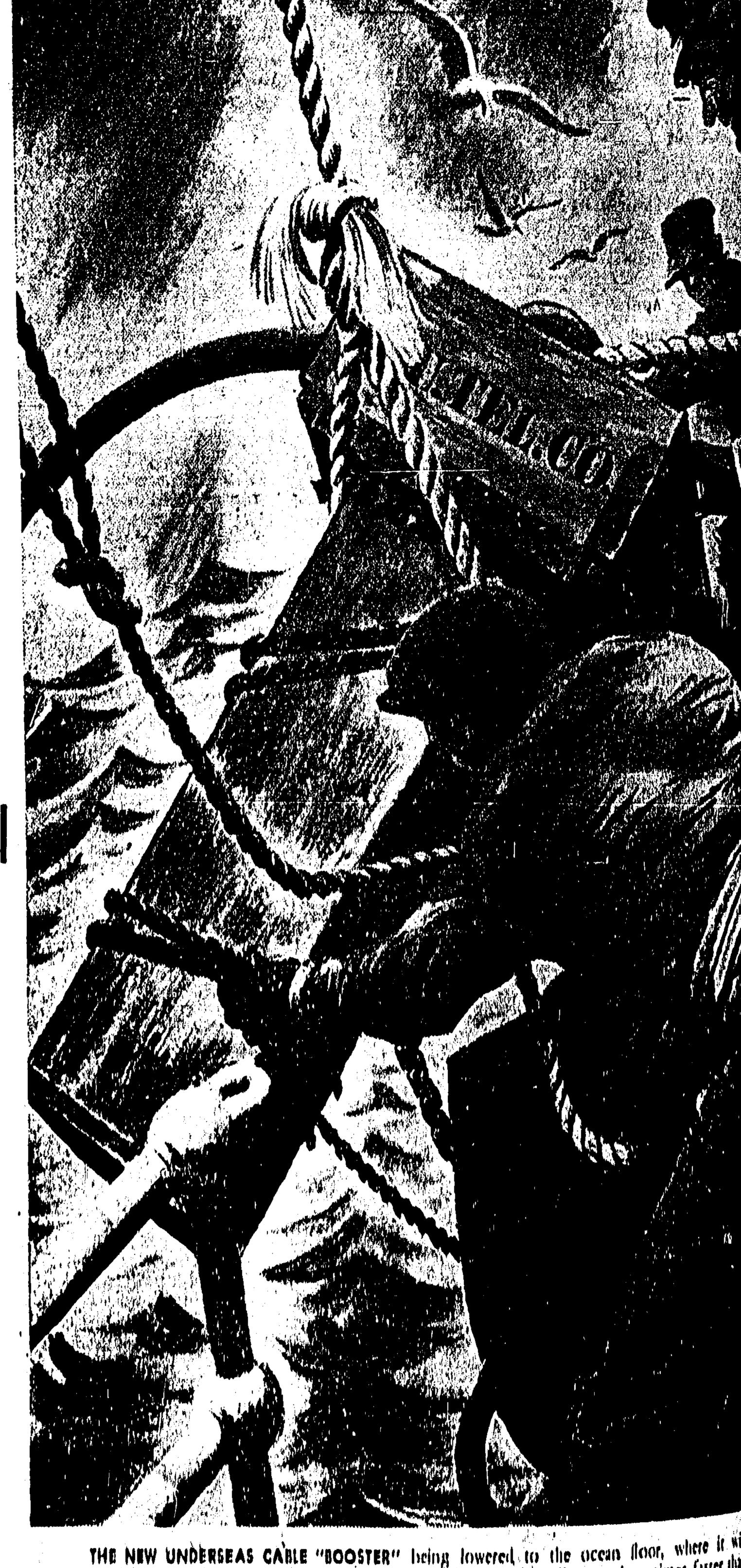
THE NEW UNDERSEAS CABLE "BOOSTER" being lowered to the ocean floor, where it willy amplify trans-Atlantic signals—allowing us to get messages from flutope three times faster than before. This is possible only because of the use of they pieces of nickel in the amplifier's vacuum toler.
