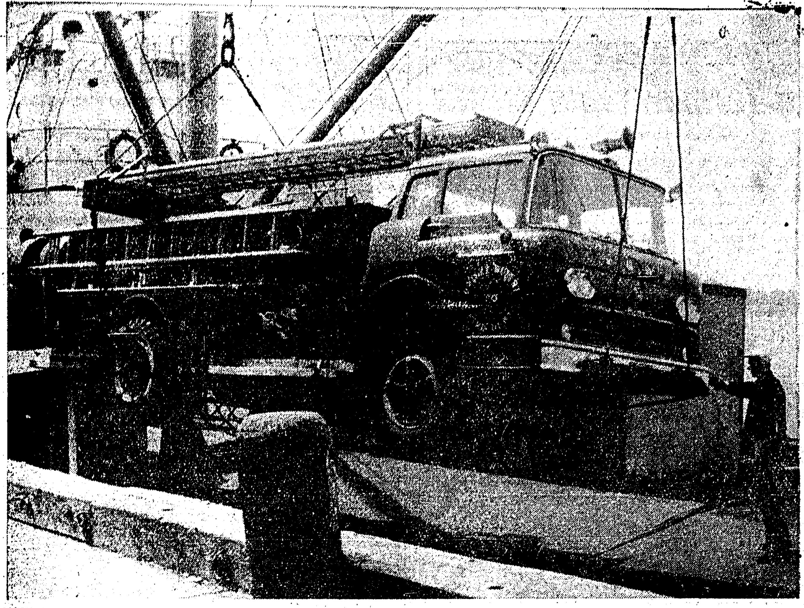
NEW FIRE TRUCK is shown above being hoisted off the Union Steamship "Cassiar" on arrival from Vancouver Friday afternoon. Truck weighs about seven tons and has a water capacity of 300 gallons. Motor, pump and body by LaFrance Company Limited is mounted on a Ford chassis.
